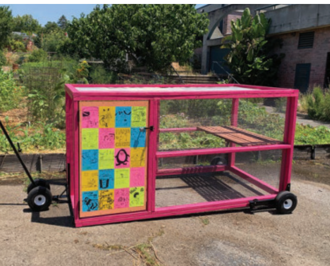
Above: Students learned how to use basic power tools, like the miter saw, drill, and impact driver, to frame and assemble the walls of the mobile chicken coops.
