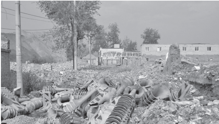
FIGURE 5.2 Jingwei School and demolition.
