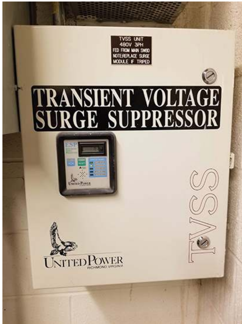
FIGURE 10.6 An industrial service entrance surge protection unit.
