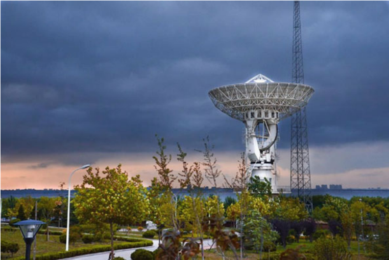
Fig. 1.2 A 18 meter in diameter reflector antenna built by the authors' team at Qingdao, China
