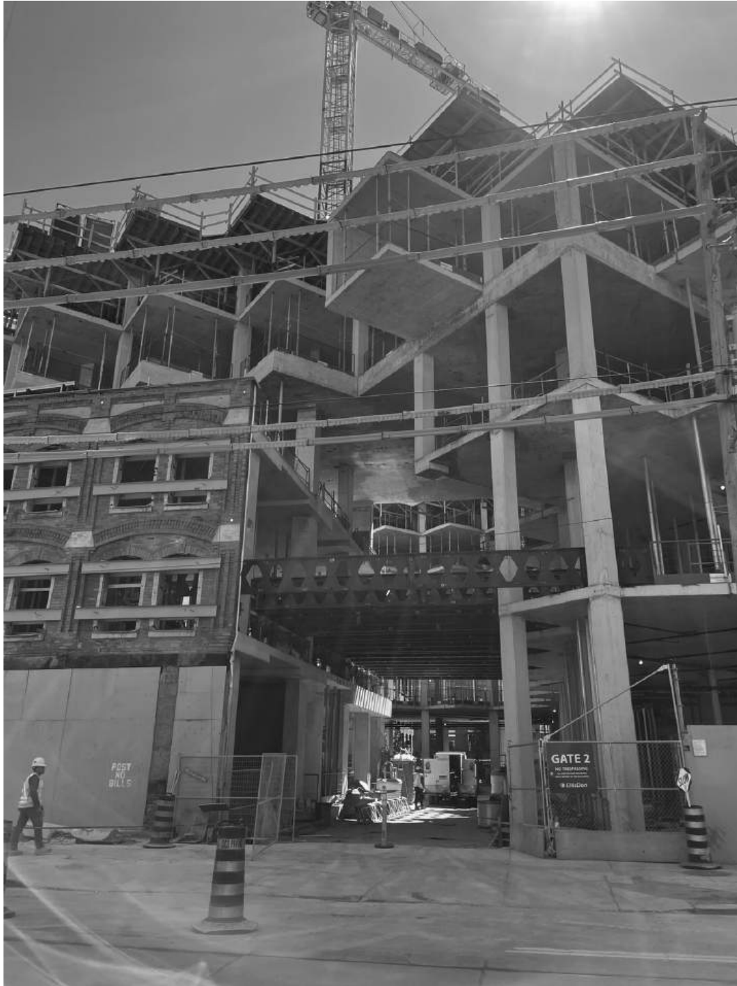
Figure 3.1.16 Construction photograph of heritage façade retention. King Toronto. Zak Fish.
