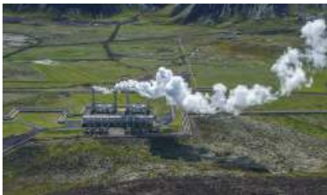
Figure 11.17 This geothermal power plant in Iceland uses geothermal energy to run steam turbines.
