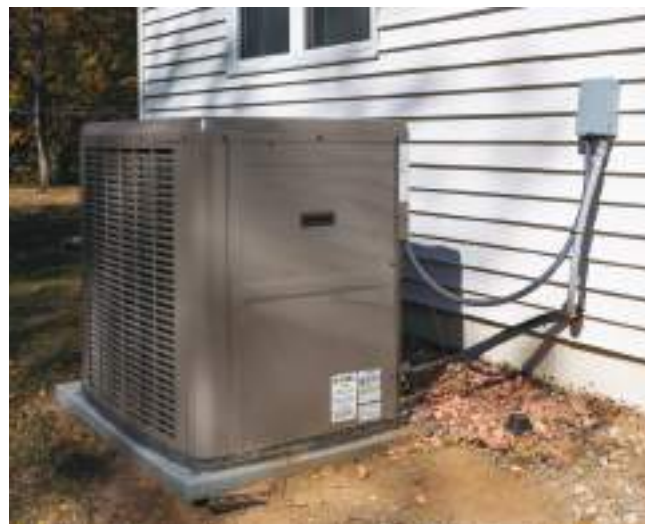
Figure 11.11 The exterior heat-exchange coils for an air-to-air heat pump are usually located behind the house or building. Mark Dierker/McGraw-Hill Education
