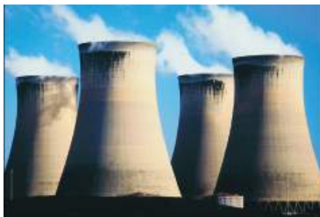
Figure 11.16 The cooling towers that are a common feature of many thermal power plants transfer heat from the cooling water to the atmosphere.
