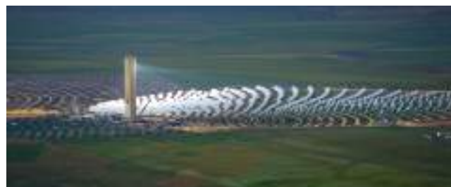
Figure 11.18 At a solar thermal power plant near Seville, Spain, high temperatures are achieved by focusing sunlight from a large array of mirrors onto a boiler located at the top of the tower.
