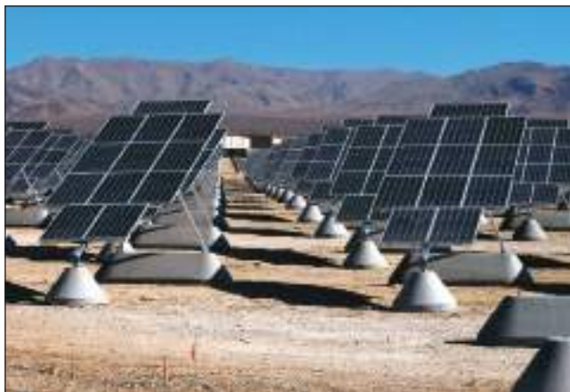
Figure 1.8 A power plant at Nellis Air Force Base utilizes photovoltaic solar cells. Stocktrek Images/Getty Images
