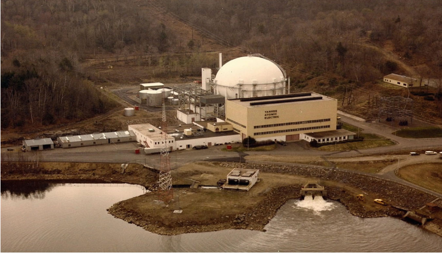
Fig. 1.1 Yankee Rowe nuclear power plant. Source Nuclear regulatory commission from US–Yankee Rowe
