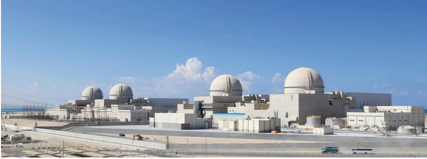
Fig. 4.2 Barakah nuclear power plant (UAE). Source Emirates nuclear energy corporation
