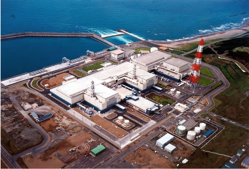
Fig. 4.1 Advanced boiling water reactor (ABWR). TEPCO Kashiwazaki-Kariwa nuclear power plant
