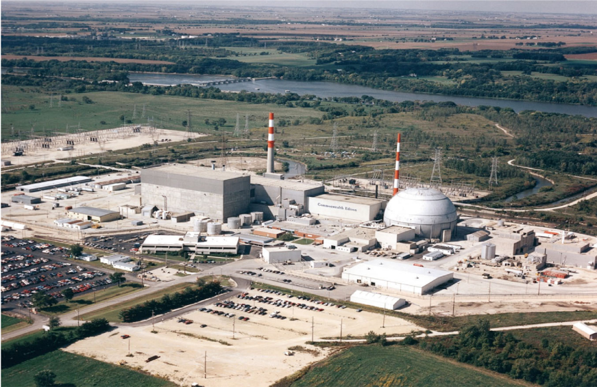
Fig. 1.3 Dresden nuclear power plants. Source NRC
