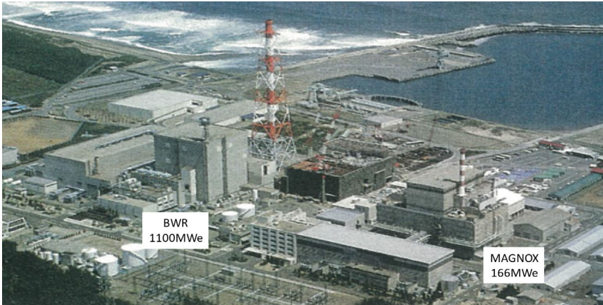
Fig. 7.1 BWR and Magnox (Graphite moderated \text{CO}_2 cooled reactor) Japan atomic Power Company, Tokaimura, Japan Source JAPC
