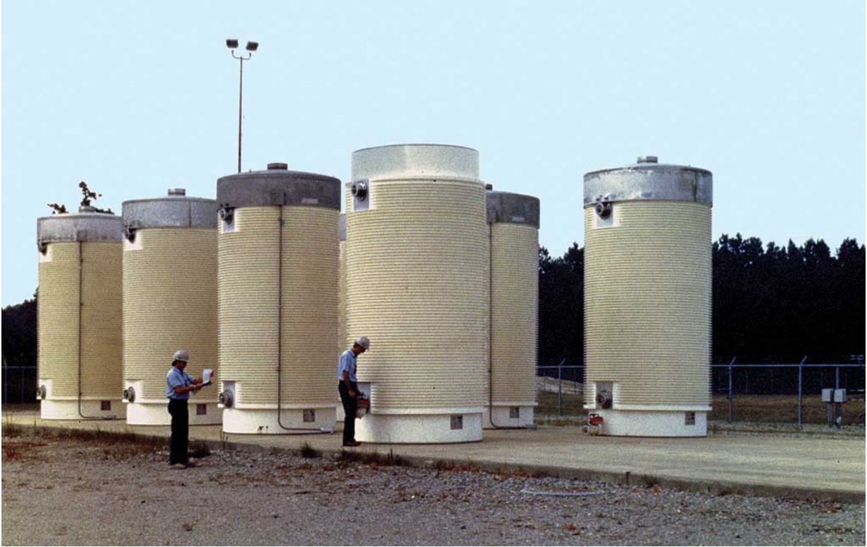
Figure 16.2 Dry storage of spent nuclear fuel in concrete casks. Reproduced from Nuclear Regulatory Commission. (2008). Wikimedia Commons. https://commons.wikimedia.org/wiki/File:Nuclear_dry_storage.jpg .
