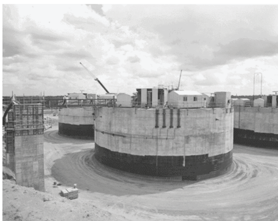
FIGURE 4.8 A 1.3 million gallon waste tank under construction. (Photo courtesy of U.S. Department of Energy.)
