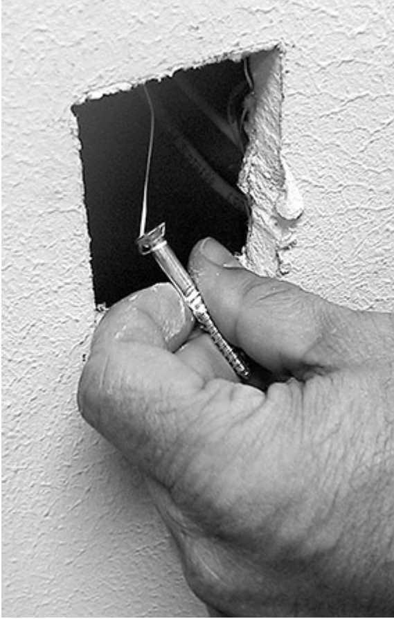
FIGURE 5-4 Dropping the cable
