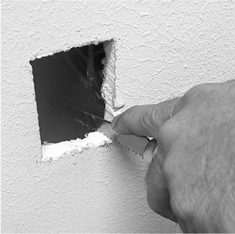
FIGURE 5-2 Cutting a hole
