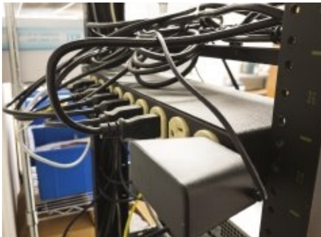
FIGURE 3.3-2 PDU in server rack
