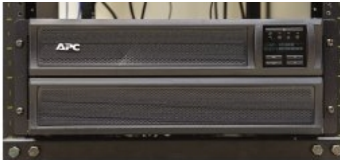
FIGURE 3.3-1 A rack-mounted UPS
