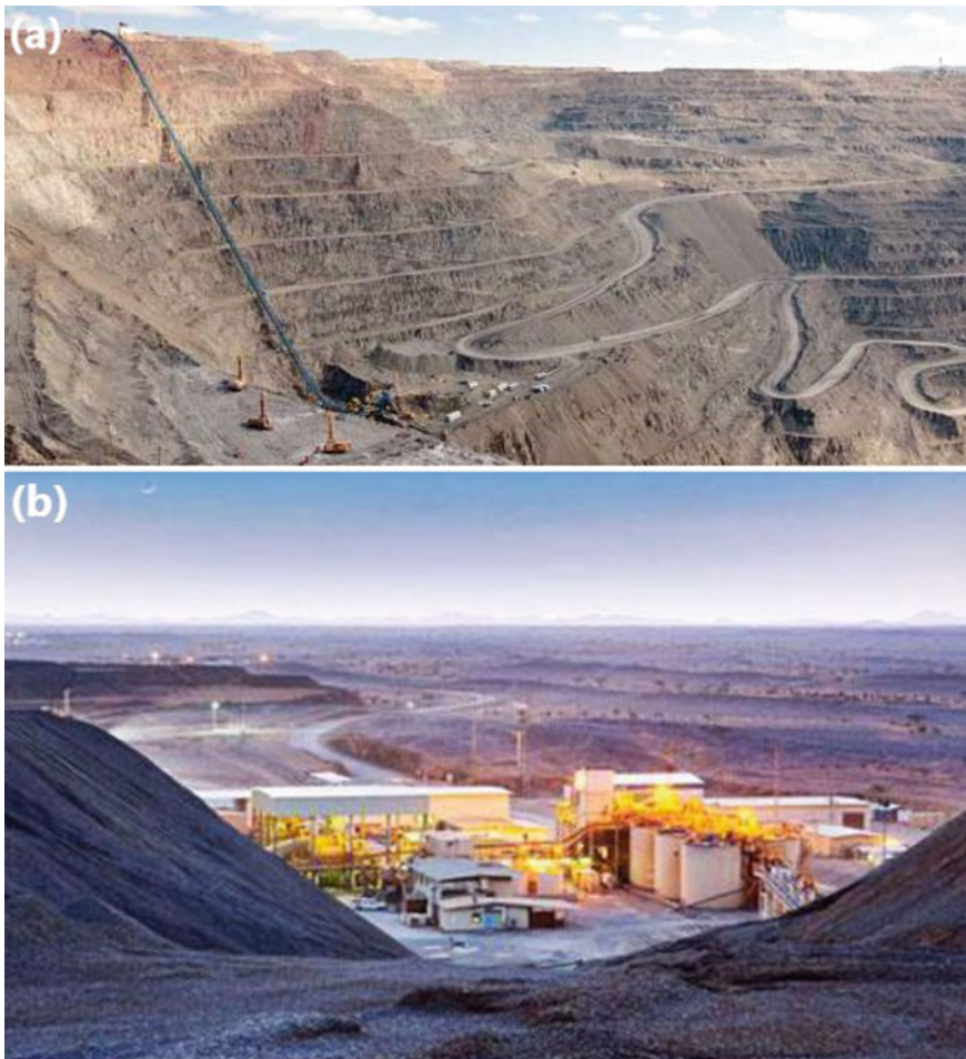
Fig 8.5 a Open-pit mine and b milling operation unite of Ad Duwayhi gold mine, southern Arabian Shield, Saudi Arabia. (Source Ma'aden Company)
