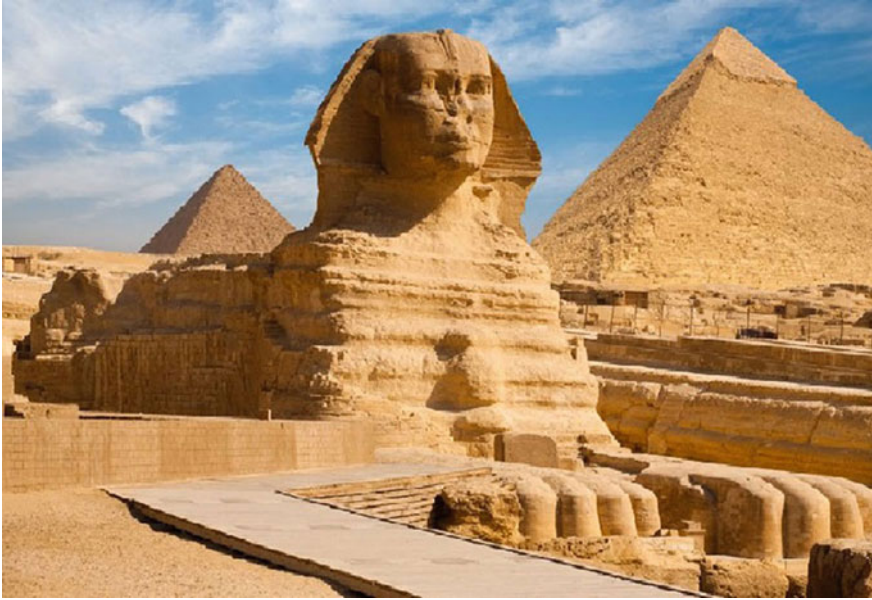
Fig. 8.17 Examples of using limestone by ancient Egyptians to build pyramids and temples. The Great Sphinx was carved from a rock in its place in the limestone quarry next to the pyramid of Khafre
