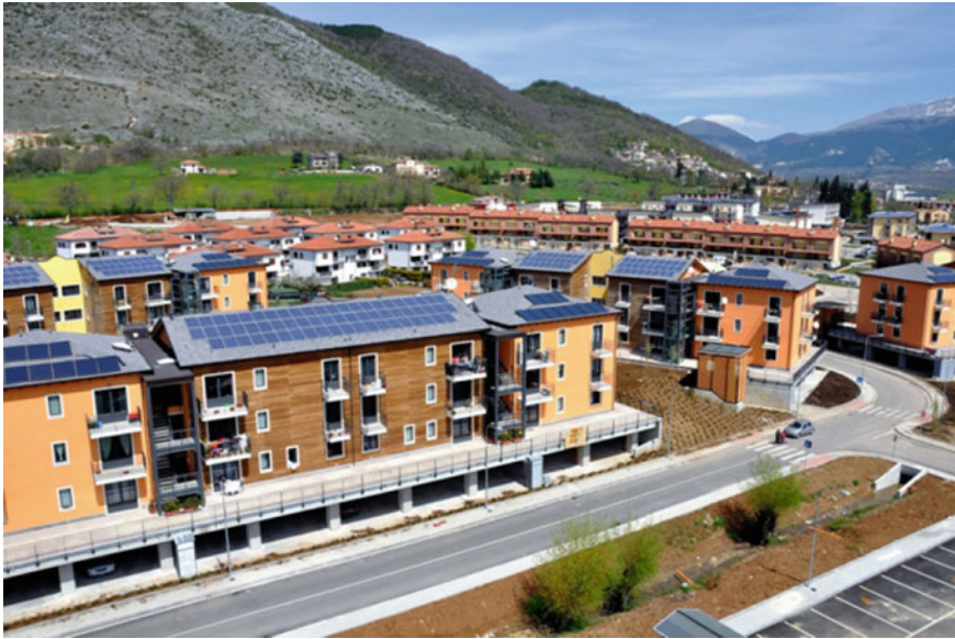
Fig. 1.15 L'Aquila C.A.S.E project. Ref. News-town, 2016
