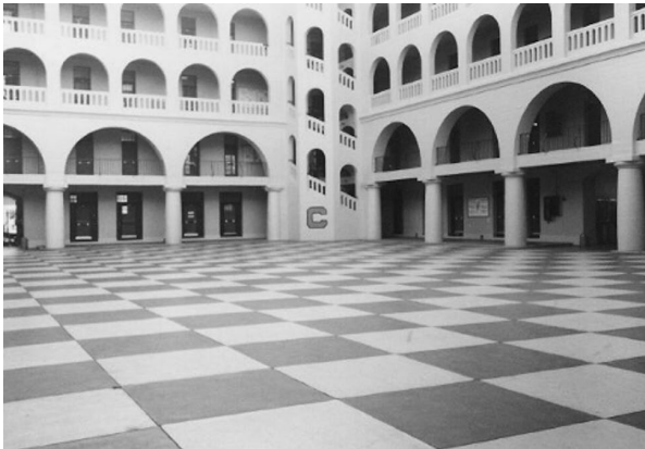
Home sweet home—the quadrangle, open-air galleries, and stairs of The Citadel’s Murray Barracks and 1st Battalion—Charlie Company
