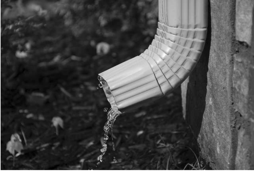
FIGURE 11.14 Short downspout too close to house.
