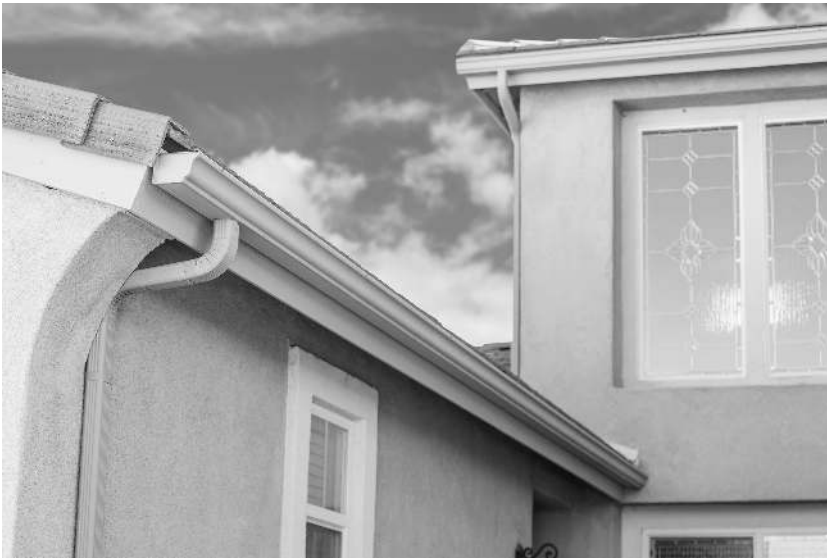
FIGURE 11.11 Extended gutter.
