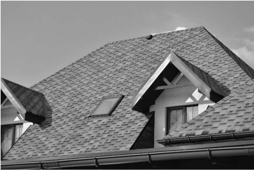
FIGURE 11.4 Hip roof.
