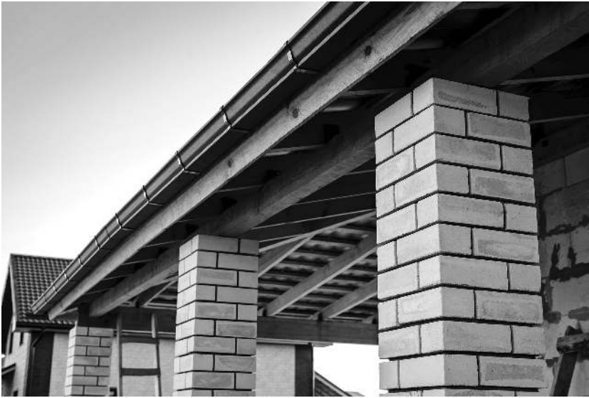
FIGURE 11.12 Extended gutter.
