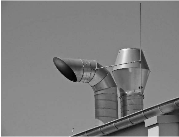
FIGURE 11.18 Exhaust points away from intake.
