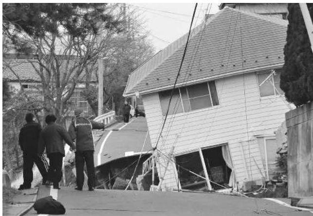
FIGURE 1.16 The damage done to a road and a house in Sukagawa city, Fukushima prefecture, in northern Japan, 11 March 2011. (Fukushima Minpo/AFP/Getty Images.)
