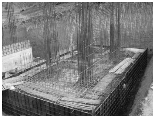
FIGURE 7.2 A raft foundation for an aqueduct under construction at 46.615 km of the Bansagar Feeder Channel, Sidhi District, Madhya Pradesh, India. (After Sanjay Kumar Shukla, Allowable Load-Bearing Pressure for the Foundation of Aqueduct on Rock/Soil at km 46.615 of the Bansagar Feeder Channel, Dist. Sidhi, MP, India. A technical report dated 7 June 2006, Department of Civil Engineering, Institute of Technology, Banaras Hindu University, Varanasi, India, 2006.)
