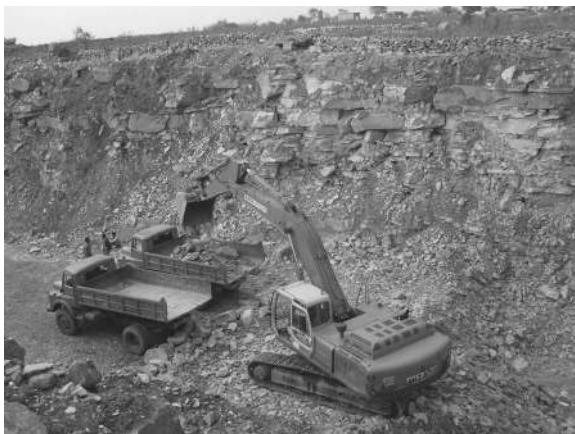
FIGURE 1.11 Heavily jointed rock mass at 0.080 km of the Meja-Jirgo link canal, the site for the construction of a canal head regulator, Mirzapur, Uttar Pradesh, India. [After Sanjay Kumar Shukla, Allowable Bearing Pressure for the Foundation Rock/Soil at km 0.080 of the Meja-Jirgo Link Canal for the Proposed Construction of a Hydraulic Structure (Head Regulator), Mirzapur, UP, India. A technical report dated 11 June 2007, Department of Civil Engineering, Institute of Technology, Banaras Hindu University, Varanasi, India, 2007.]
