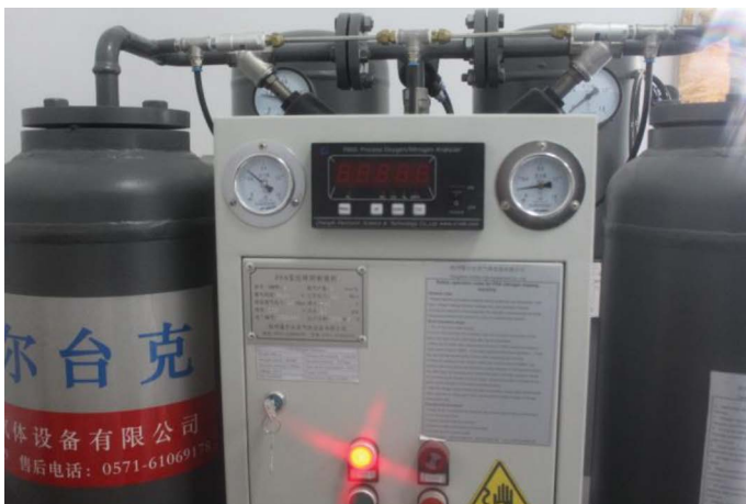
FIGURE 7.3 Inert gas supply of nitrogen.
