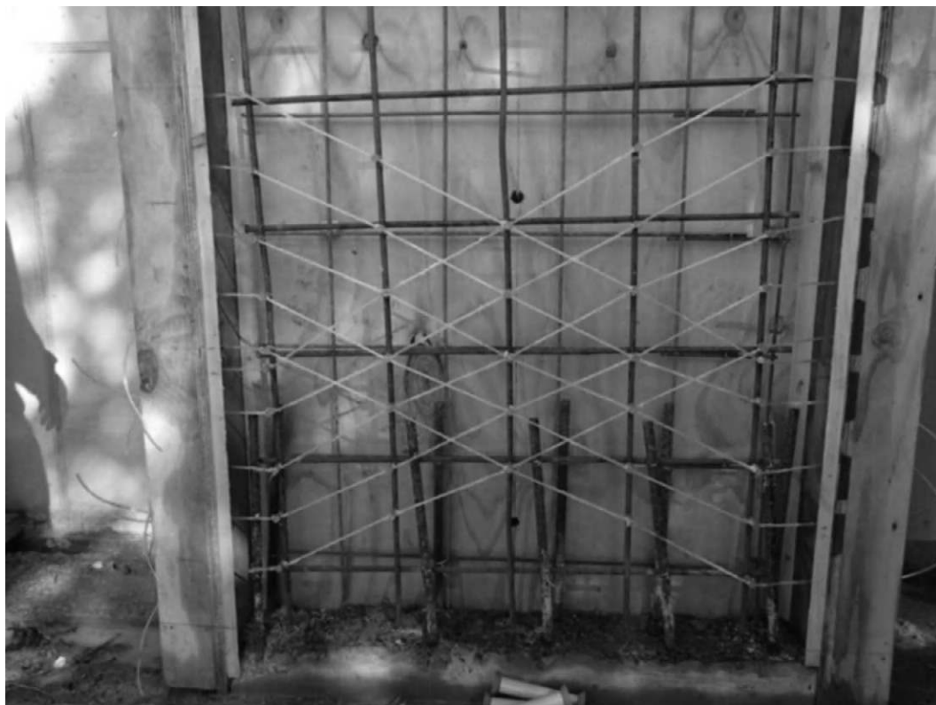
FIGURE 7.16 Vascular system for providing nutrients to bacteria-based self-healing of concrete in diagonal tubes placed in formwork. (From [Paine 2016].)
