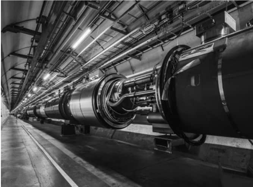
FIGURE 13.4 LHC SC magnets in the underground tunnel. Source: CERN
