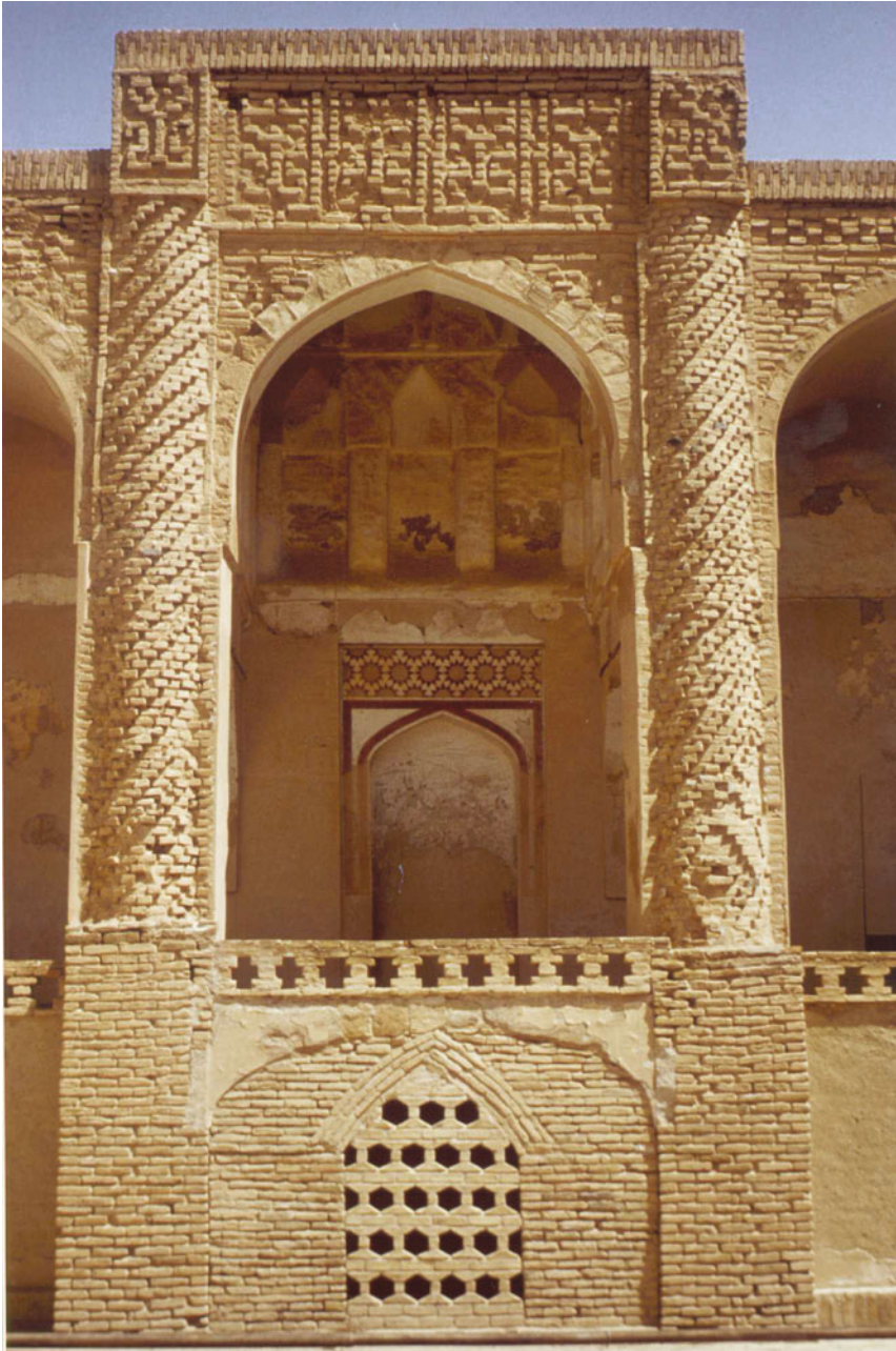
Illus. 3.4.2 Brick ornaments at the Iwan of the Friday Mosque of Nain, Iran. An Iwan (also Eiwan or Liwan) is the overarching porch of a prayer room, which is opened towards a yard with its narrow side
