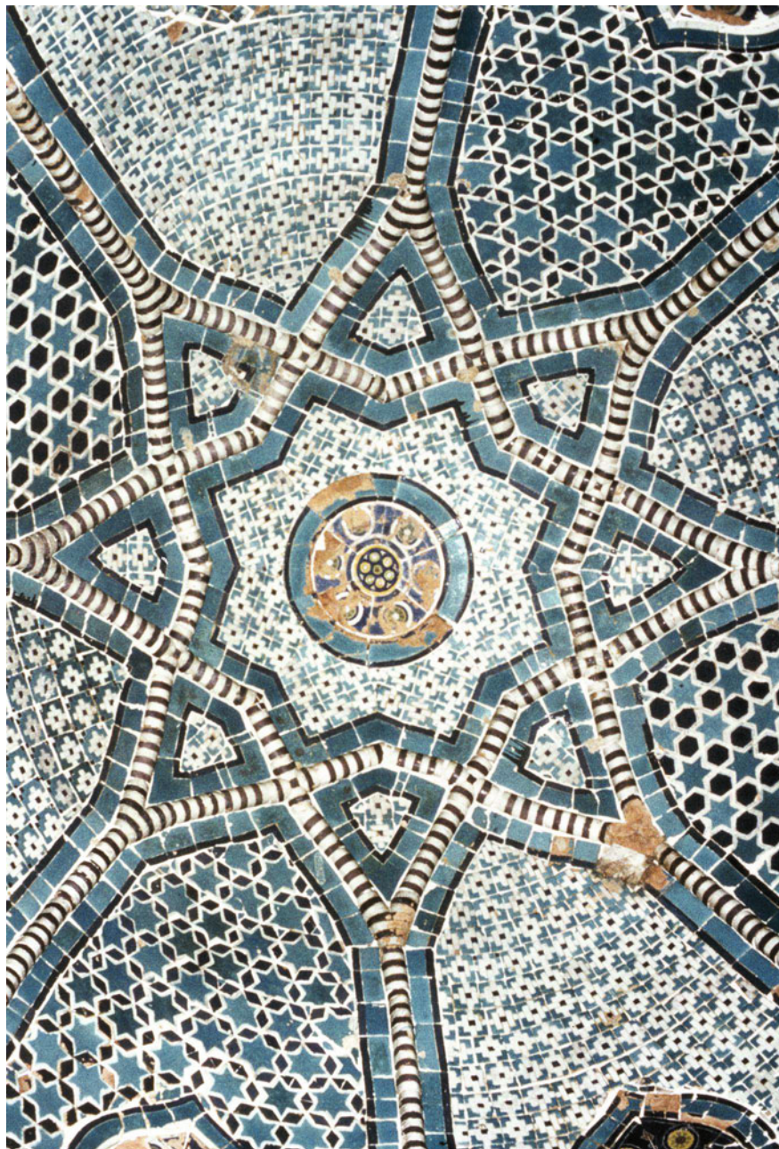
Illus. 3.4.6 Dome decoration of a Mausoleum in Shah-i Zinda, Uzbekistan [Photo: H.-W. Alten]
