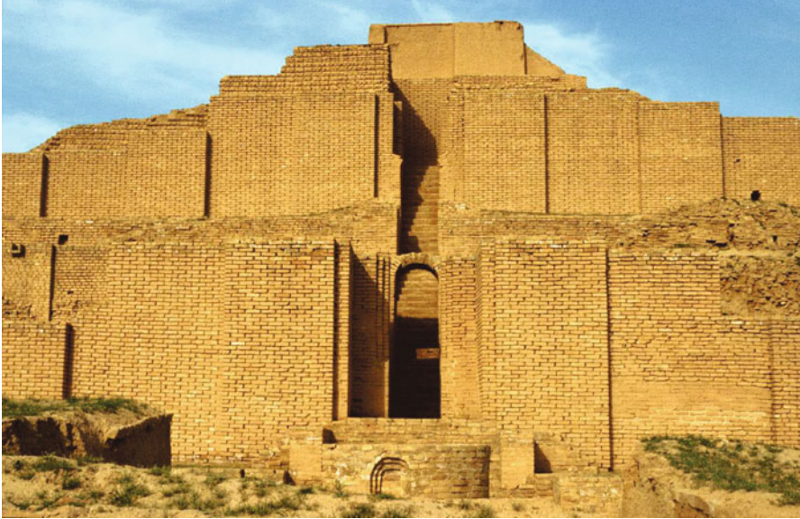
Illus. 1.2.7 Ziggurat of Chogha Zambil. The gradual tower made of clay bricks has the typical shape of a temple erected by the Sumerians, Babylonians, Assyrians and Elamites. The five-stage Ziggurat of Chogha Zambil built around 1250 BC is the best preserved building of its kind
