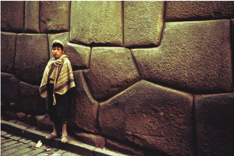
Illus. 3.5.15 Cyclopean wall in Cuzco (Perú). The Incan master builders designed true marvels of precision with these walls made of gigantic, polygonal stone blocks in the capital of the Incan Empire.
