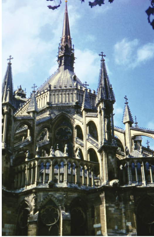
Illus. 4.4.4 Apse of the Cathedral Notre Dame of Reims, France. In his sketchbook Villard d' Honnecourt has adhered the design of buttresses and their pinnacles [Photo: H.W. Alten]
