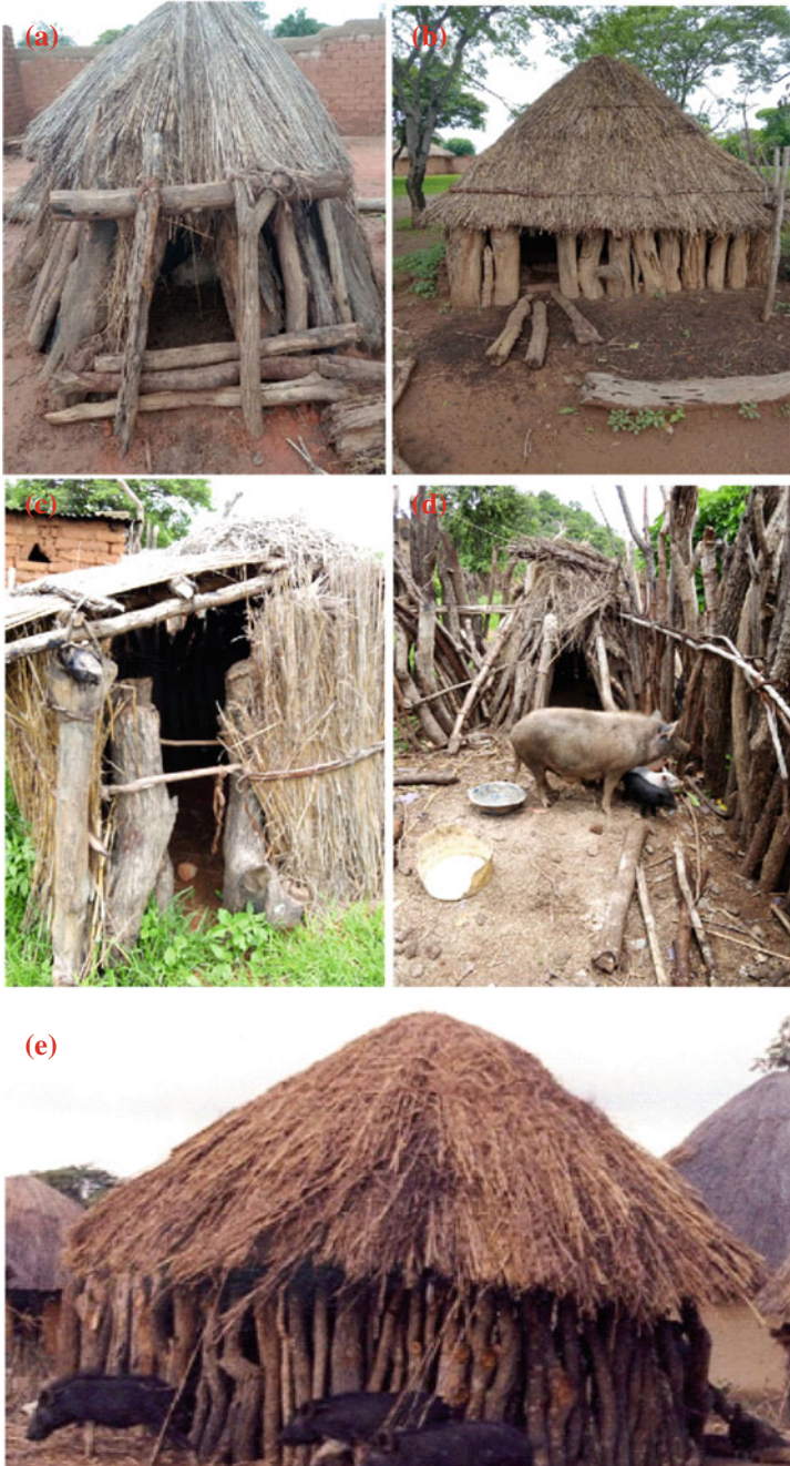
Fig. 2 Types of pig kraals: a-e are mainly constructed using wooden poles and trusses, grass thatch roofs, bare or covered by iron sheets. Floors are earthen. Sources Sinda and Katete districts of eastern province of Zambia
