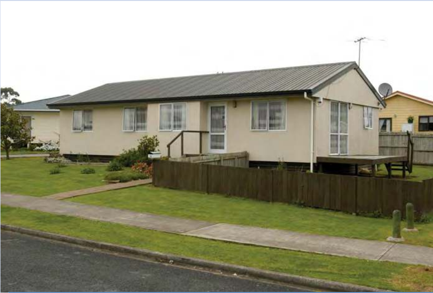
Figure 8.1 The house built in fewer than four hours. Source: Photo courtesy of Habitat for Humanity.
