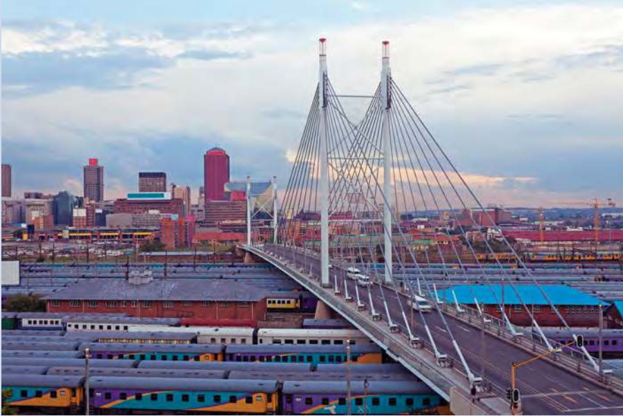
Figure 11.10 Nelson Mandela Bridge, Johannesburg.
