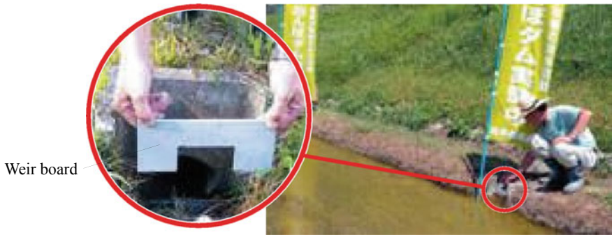
Fig. 5.3 Paddy field dam. Source Modified from the Ministry of Agriculture, Forestry and Fisheries of Japan, https://www.maff.go.jp/j/nousin/noukan/nougyo_kinou/pdf/adult_zentai.pdf , Accessed October 31, 2021 (in Japanese)
