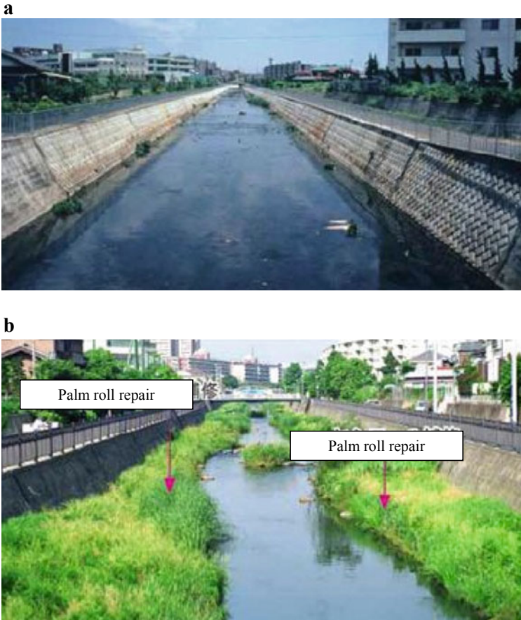
Fig. 6.10 Example of nature-oriented river construction in the Itachi River in Yokohama City; a before construction and b after construction. Source Modified from the National Institute for Environmental Studies, https://tenbou.nies.go.jp/science/description/detail.php?id=95 , Accessed October 31, 2021 (in Japanese)
