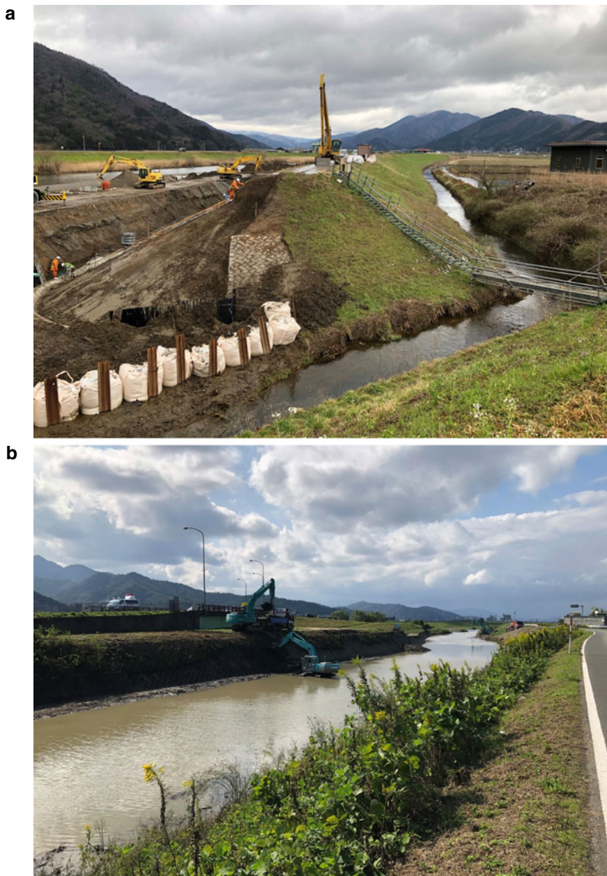
Fig. 2.8 Strengthened embankments ( Photos by Akira Matsui ). Notes The photos were taken at an open levee. a The photo was taken at the confluence between the Onyu River and Kita River. Photo date: February 26, 2021. b The photo was taken at the confluence between the Nogi River and Kita River. Photo date: October 14, 2020
