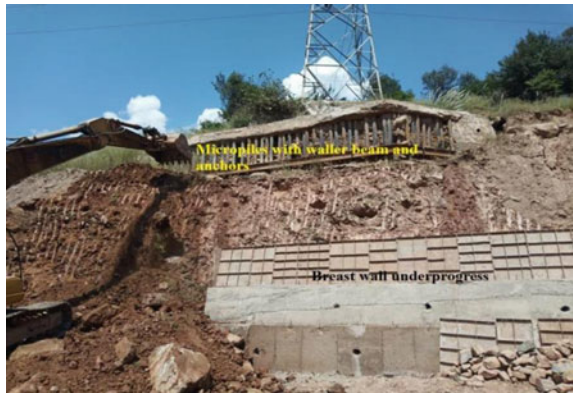
Fig. 3 Typical section of micro-piling for tower protection
