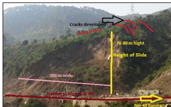
Photograph 3 Samroli landslide with dimension and cracks marked, during Sept. 2016 event
