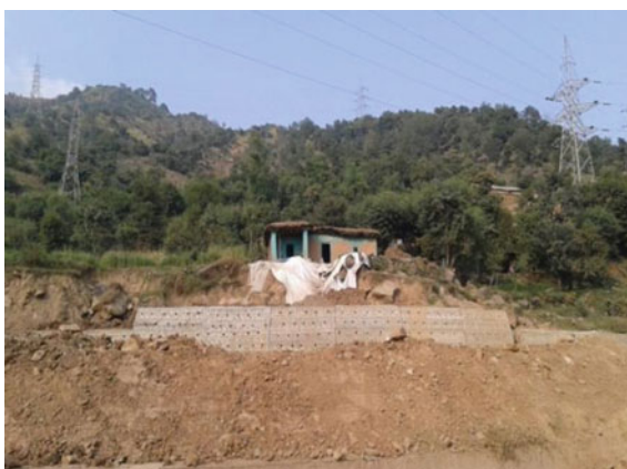
Photograph 8 House damage and geological strata near the ROW at Bali village
