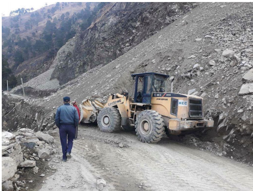
Fig. 3 Landslide at study area triggered due to the heavy rainfall during year 2019 (25-02-19)
