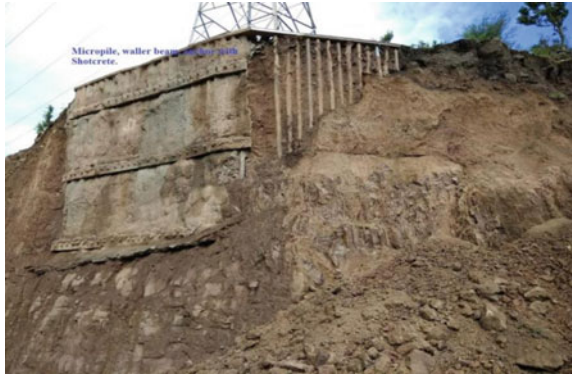
Photograph 17 Tower protection with micro-pile and breast wall in study area
