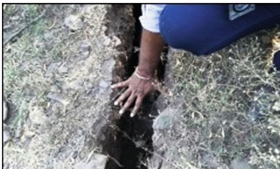
Photographs 4 Cracks developed at top of Samroli slide during September 2016 event
