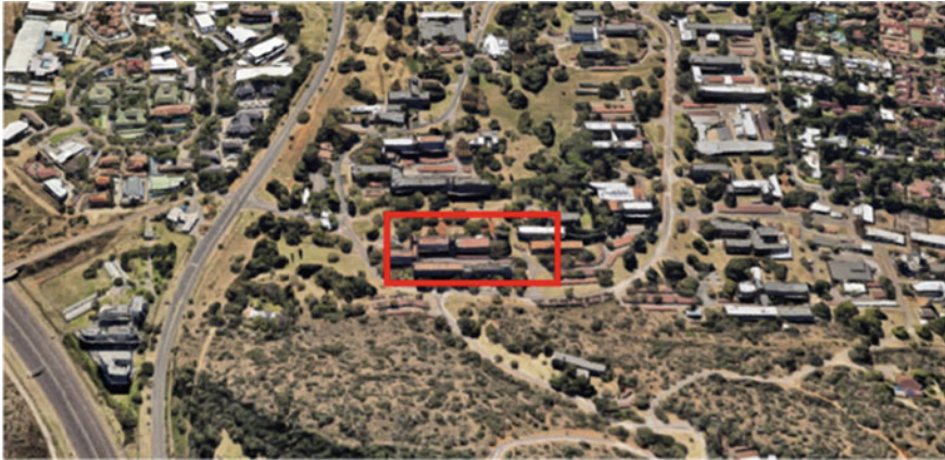
Fig. 2 Aerial photograph of the building and site
