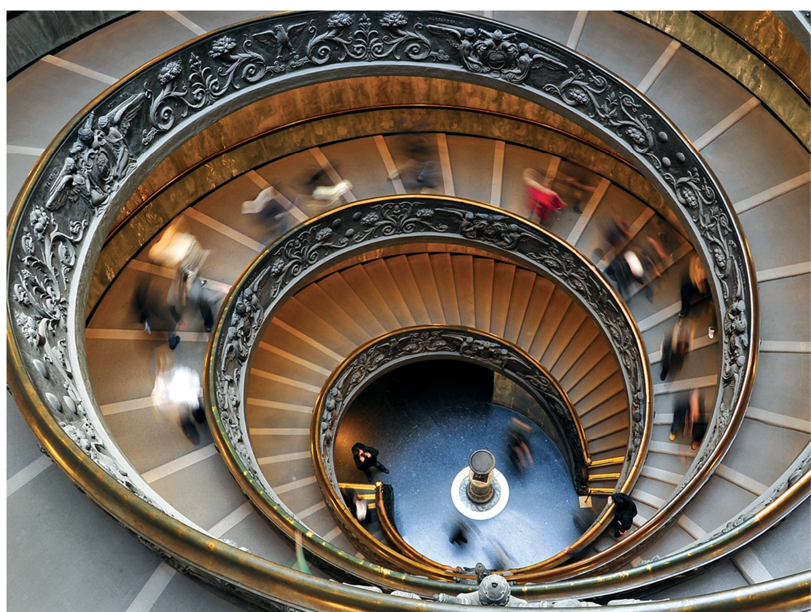
The double spiral staircase at the Vatican Museums (p. 94), inspired by a 1505 design by Bramante, allows visitors to pass in both directions without encountering one another.
