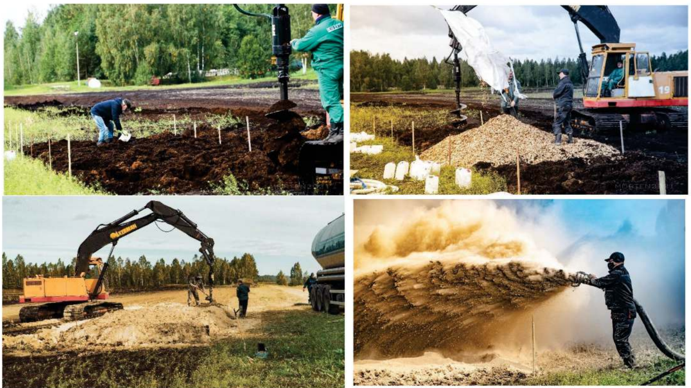
Figure 3. Clockwise from top left: preparatory work in Sangla bog; adding components; spreading of oil shale ash; road surface leveling.
