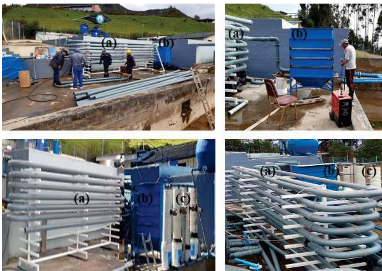
Figure 13. Implementation of the Pilot Treatment System. The upper left figure shows the HTF implementation; in the upper right, the implementation of the settler is presented. The complete experimental system is presented in the lower left and right figures, as follows: (a) HTF, (b) high-rate settler, and (c) rapid sand filters.
