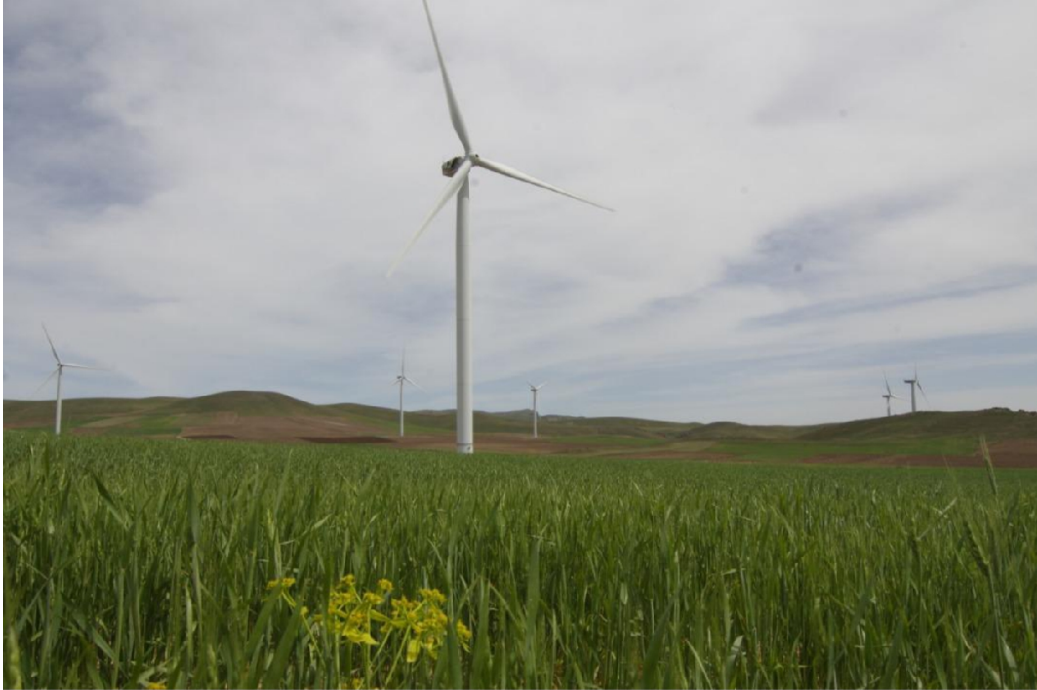
(a) Mapna 2.5 MW turbines used in Aghkand farm
