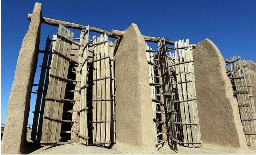
FIGURE A.2 The rotor of Nashtifan's windmills.
