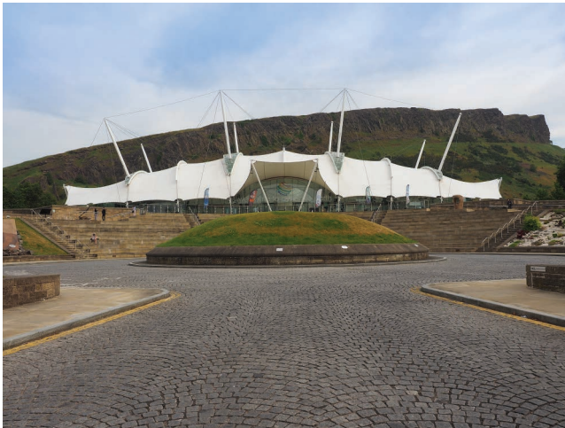
FIGURE 8.3 Dynamic earth, Edinburgh, showing its tensioned membrane roof structure. (Source: Shutterstock.)
