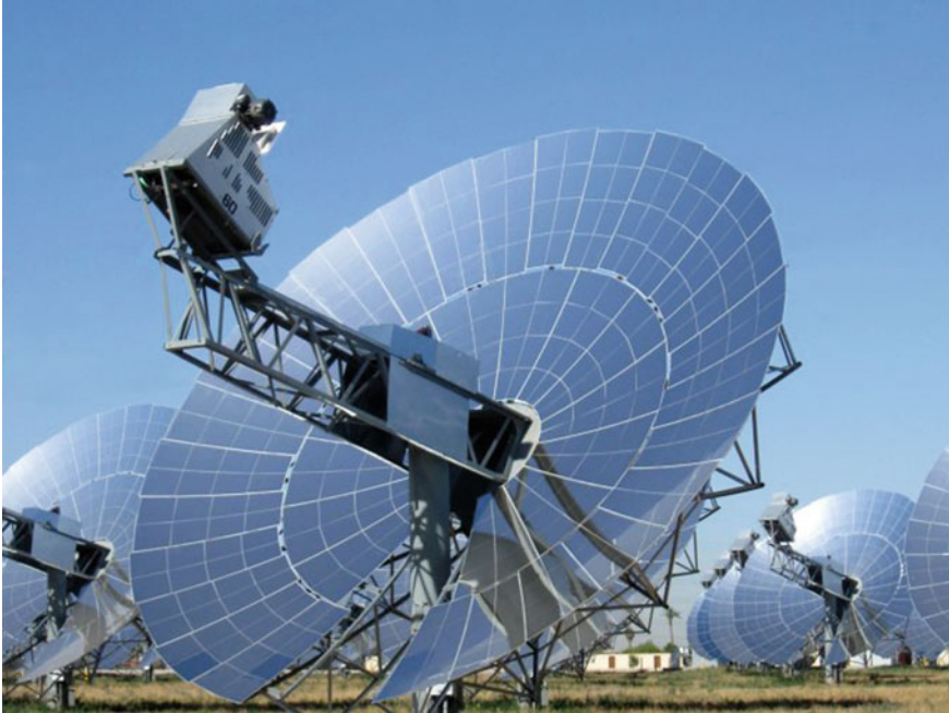
Fig. 8.3 Solar thermal power plant with big dish concentrator [7]
