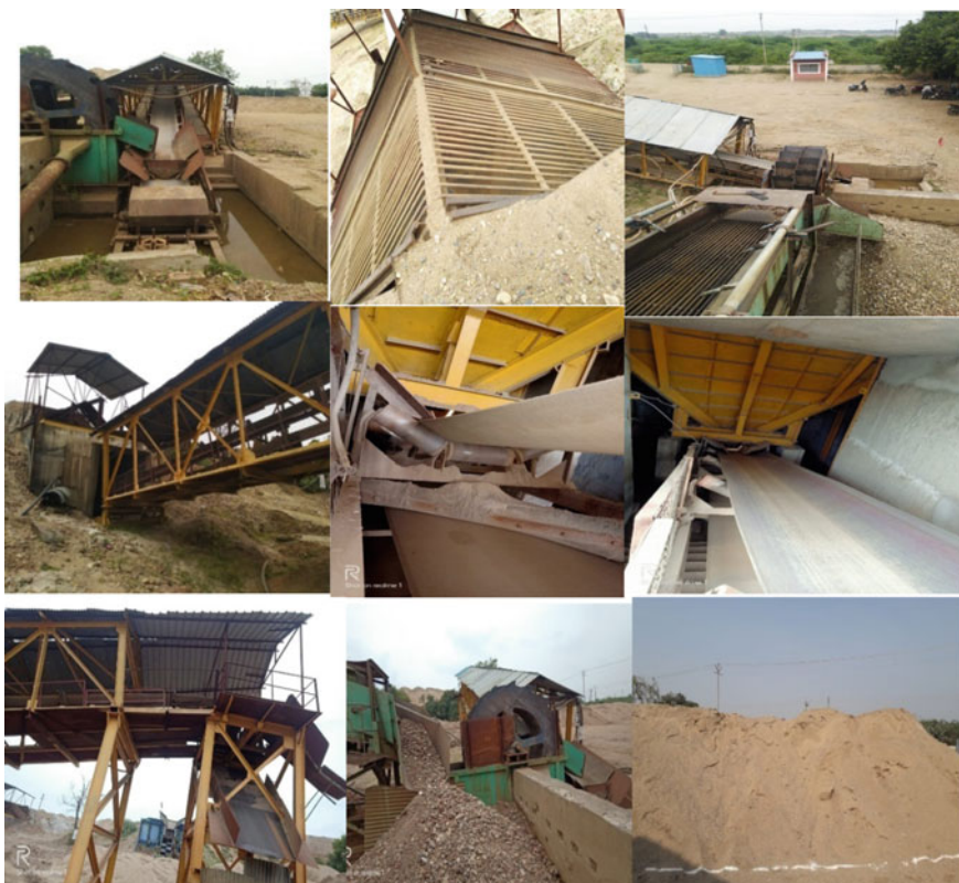
Fig. 4 Components of segregation plant
