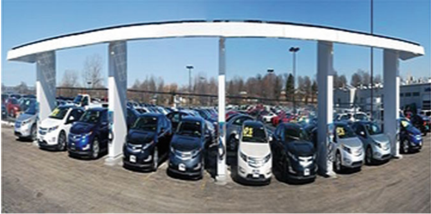
Fig. 6 A solar powered charging station
