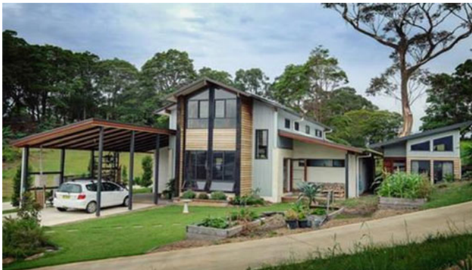
Fig. 8 Hemp house in Mullumbimby designed by Barefoot sustainable design [24]
