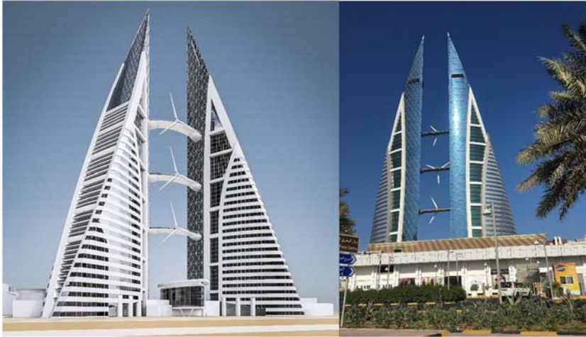
FIGURE 6.2 Bahrain world trade center; left schematic front view and right: real photo from behind [8].
