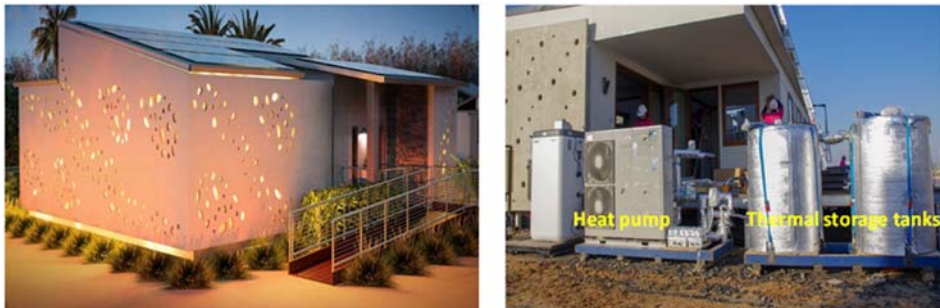
FIGURE 2.10 Illustration of the case study building, heat pump, and thermal storage tanks.
