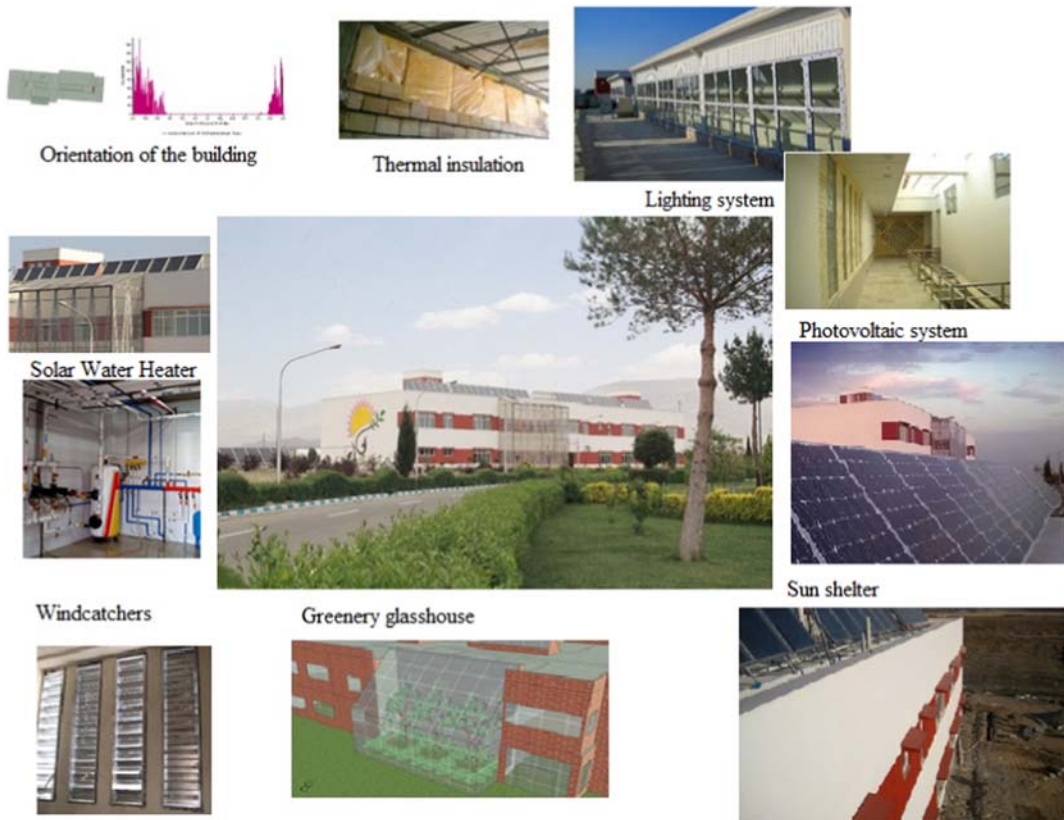
FIGURE 6.9 Solutions for reducing energy consumption in the NZEB in the Materials and Energy Research Center located in Tehran, Iran.
