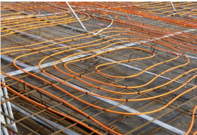
FIGURE 10.13 Thermal slabs during installation under the first floor of the building.
