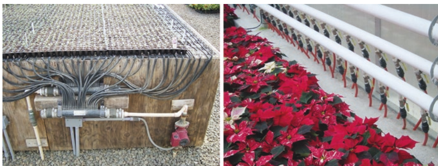
Fig. 11.4 Examples of root-zone heating systems: bench heating (left, heating tubes installed between the bench surface and the bottom of the seedling flats) and floor heating (right, heating tubes embedded in the concrete floor). (Photographs by A.J. Both)
