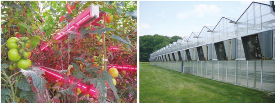
Fig. 11.2 Examples of supplemental lighting (left; using light emitting diodes) and mechanical ventilation (right; using electric-driven exhaust fans) used in greenhouse operations. (Photographs by A.J. Both)
