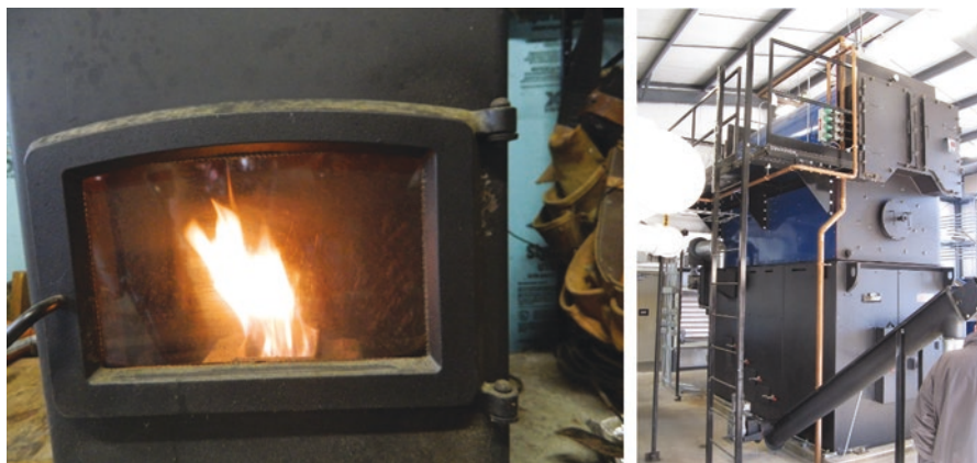
Fig. 13.4 Pellet stoves (left) provide a reliable, low maintenance source of heat, relying on densified biomass. Commercial wood boilers (right) are an efficient option for farms with larger heating loads. (Photos by EV Johnstonbaugh, D Ciolkosz)
