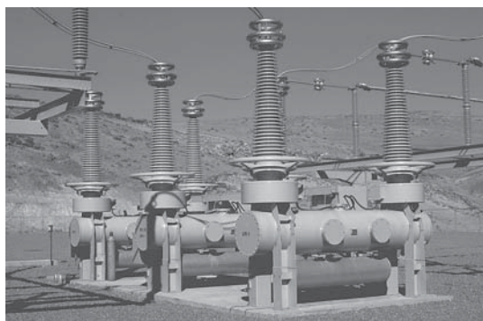
Figure 4-28 161-kV gas breaker.
