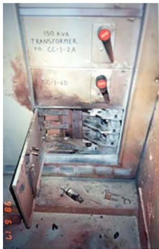
Figure 11-13 Arc flash. IEEE Std 1584-2018/IEEE.
