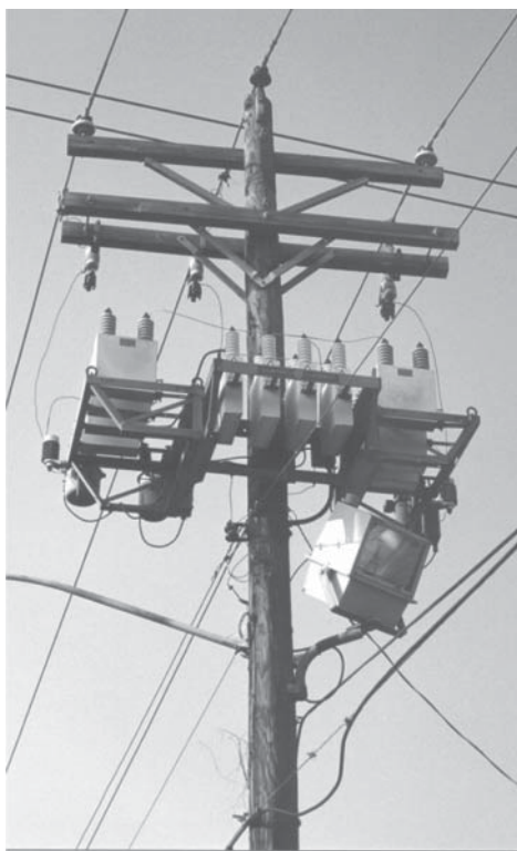
Figure 4-43 Station capacitor bank.
