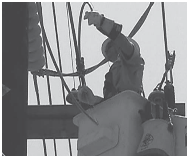
Figure 11-11 Live maintenance distribution.
