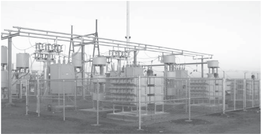
Figure 4-47 Static VAR compensator.
