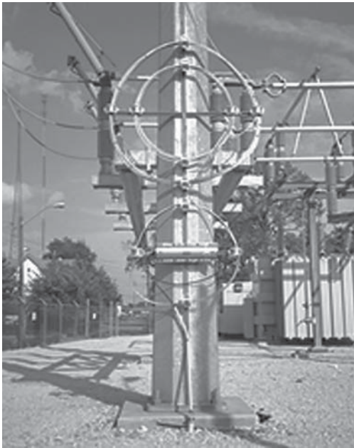
Figure 9-6 Substation optical fiber cables.
