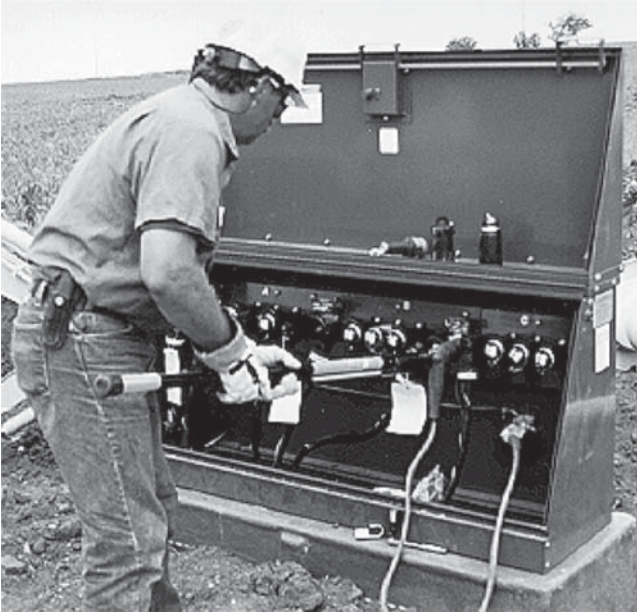
Figure 5-32 Load break connections.
