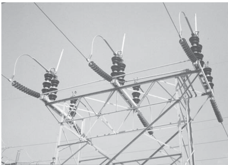
Figure 4-36 Vertical air disconnect switch.
