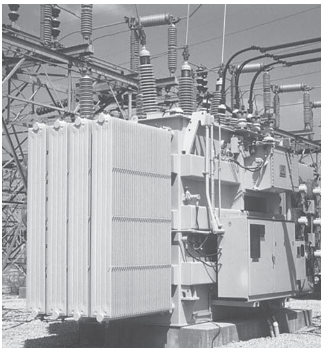
Figure 4-2 Distribution power transformer.
