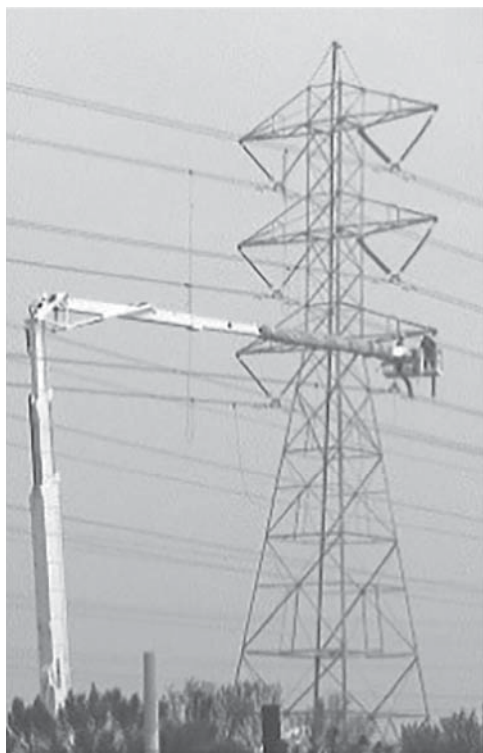
Figure 11-7 Insulated buckets.
