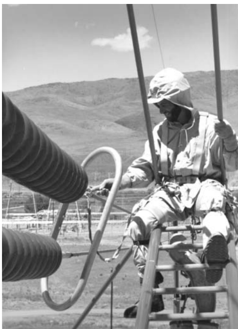
Figure 11-9 Bare hand live line maintenance.
