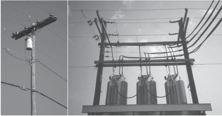
Figure 4-3 Transformer bank.
