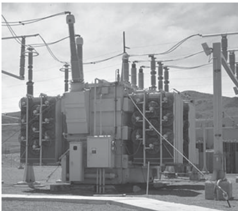
Figure 4-1 Step-down transformer.
