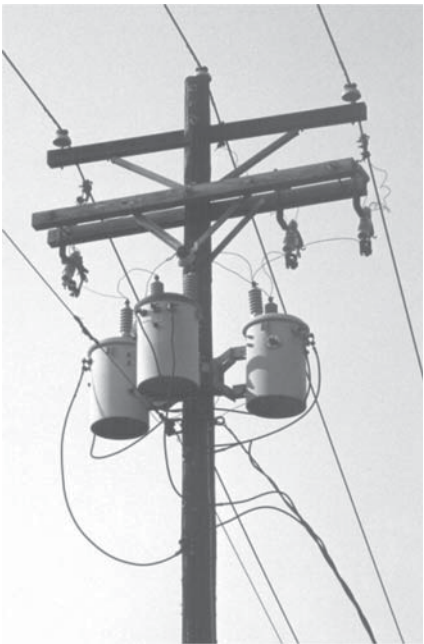
Figure 5-19 Three-phase transformer bank.
