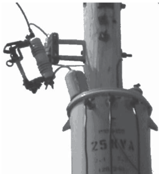
Figure 5-26 Fuse cut-out.
