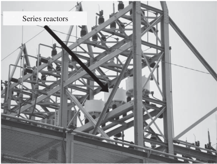
Figure 4-46 Series reactors.
