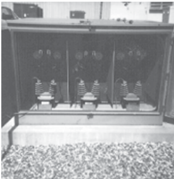
Figure 6-11 Underground primary metering.
