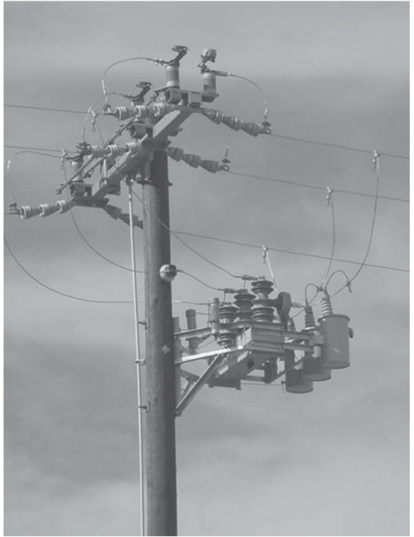
Figure 6-12 Overhead primary metering.
