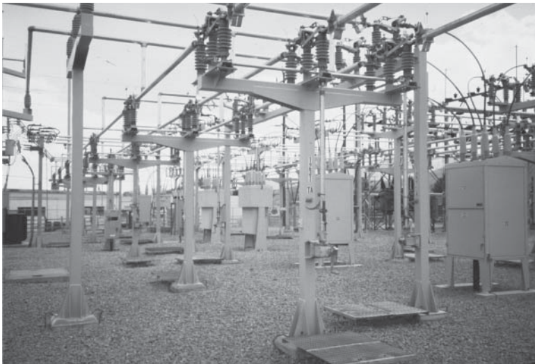
Figure 4-42 Example of typical electrical bus.
