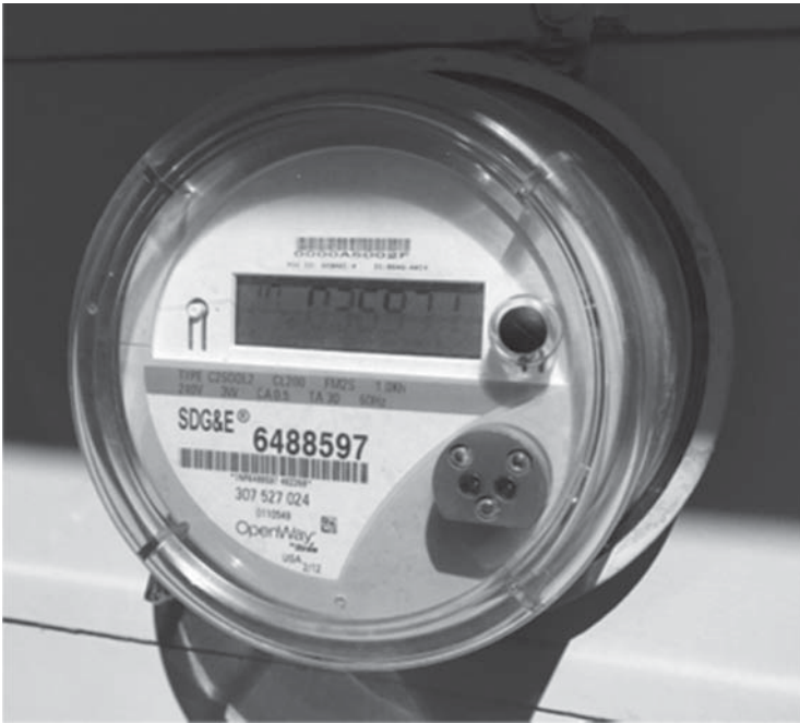
Figure 6-9 Residential smart meter.
