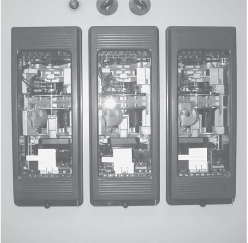
Figure 7-2 Electromechanical relays.
