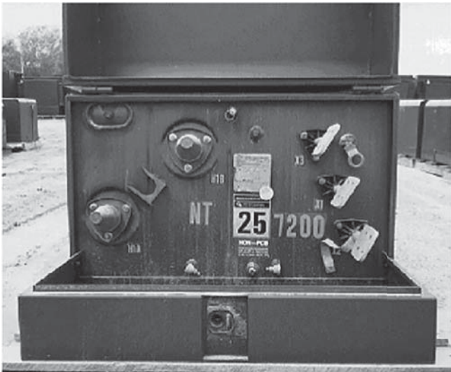
Figure 5-37 Loop transformer.
