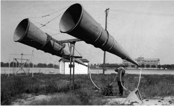
Figure 1.2 Aircraft engines produced unprecedented sound, so in order to hear them at a distance, the war efforts developed listening devices. A two-horn system at Bolling Field, USA, 1921. Sound location equipment sometimes had four acoustic horns, a horizontal pair and a vertical pair, connected by rubber tubes to stethoscope type earphones worn by two technicians that enabled one to determine the direction and the other the elevation of the aircraft. Source: Unknown author/Wikimedia Commons/Public Domain.
