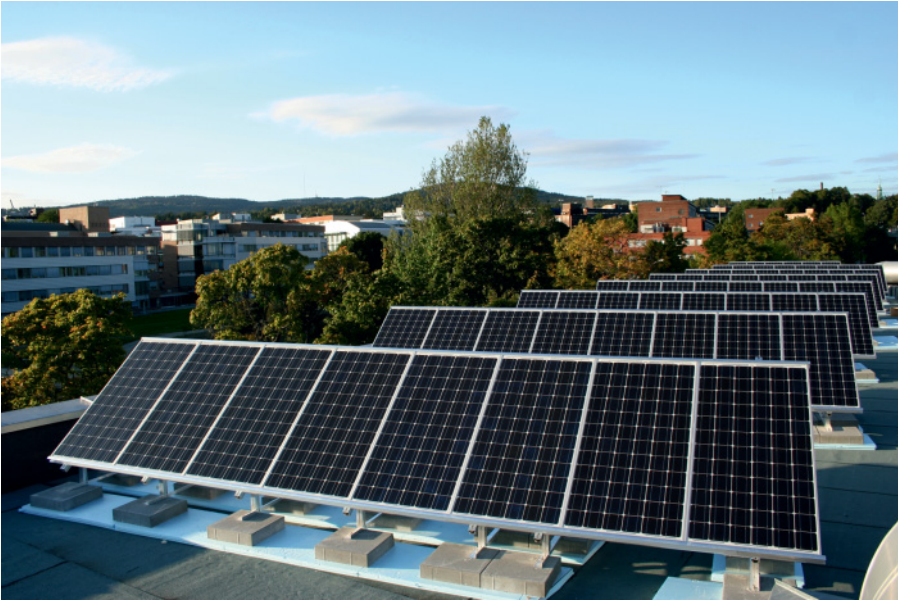
Figure 4.2 Raising the power level: a 17.6kW p grid-connected roof installation on the Oslo Innovation Centre, Norway (IEA-PVPS).
