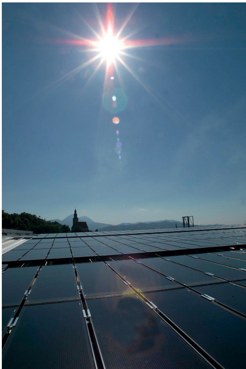
Figure 2.29 An array of CIS solar modules in Austria (EPIA/Shell Solar).
