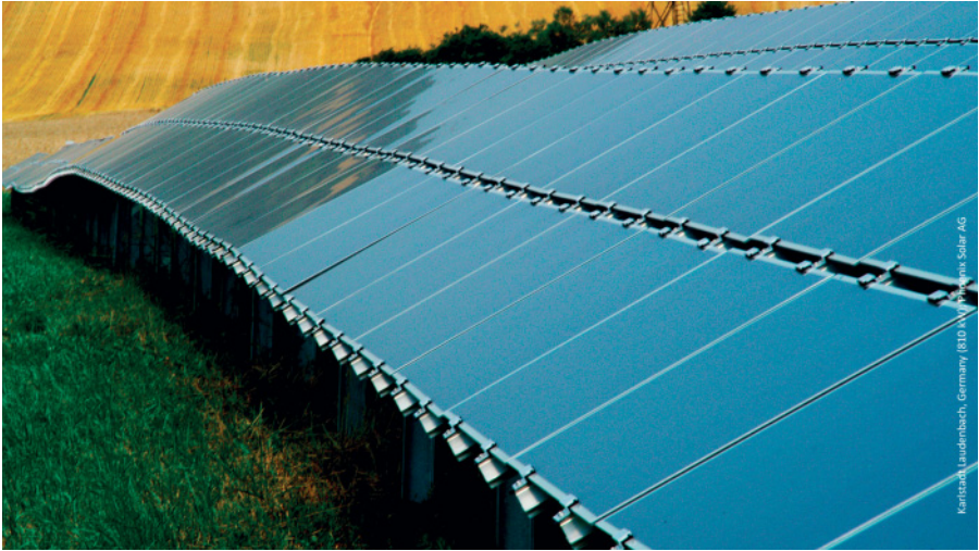
Figure 2.31 Farming the Sun: part of an 810 kW p CdTe power plant in rural Germany (First Solar/Phoenix Solar).
