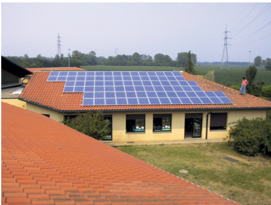
Figure 1.13 A 9kW grid-connected PV system in Northern Italy (IEA-PVPS).
