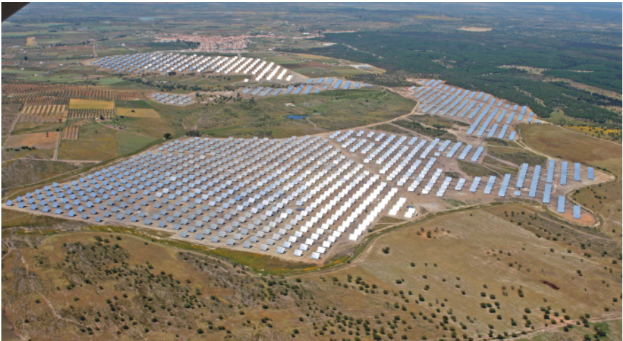
Figure 4.6 The Moura power plant in Portugal, rated at 45.6MW p , represents a big challenge for inverters as well as PV cells and modules (IEA-PVPS).
