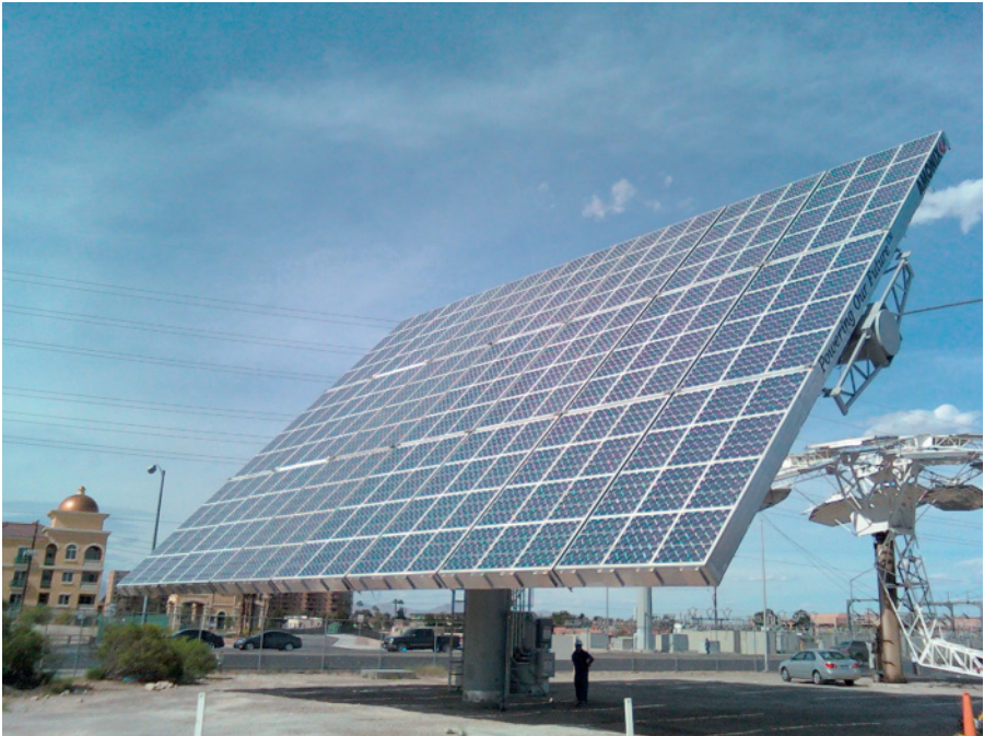
Figure 3.21 This impressive two-axis tracker in Las Vegas, USA, supports multiple point-focus concentrator modules housing multijunction GaAs solar cells and is rated at 53\text{ kW}_p (Amonix Inc.).
