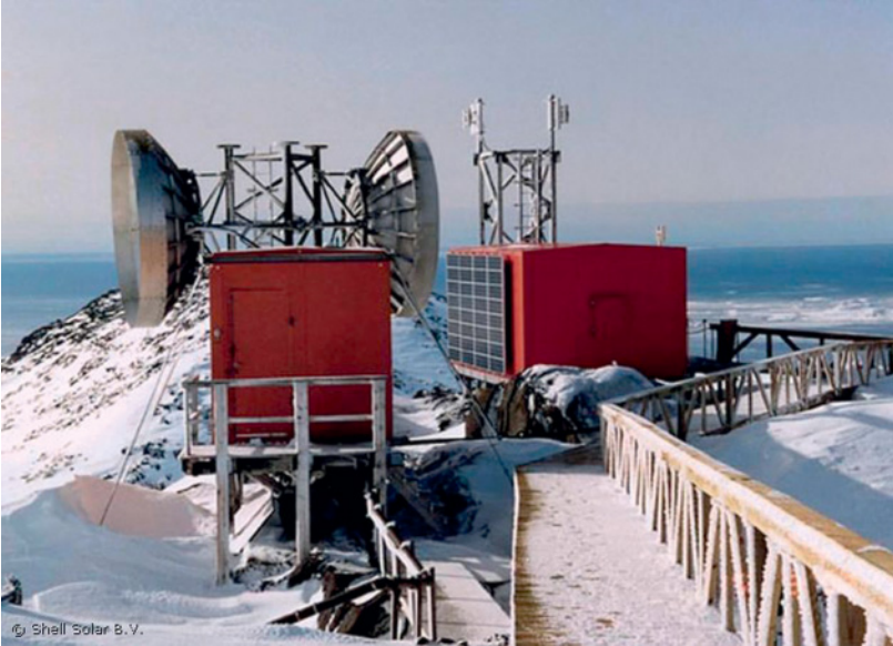
Figure 5.35 A PV array produces electricity for a meteorological station in Greenland. In this high northern latitude the vertical array captures much of the available sunlight, and solar cell efficiency is enhanced by the very low temperatures (EPIA/Shell Solar).
