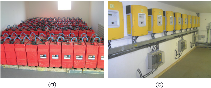
Figure 5.24 The battery banks, and some of the main inverter-chargers (Wind & Sun Ltd).
