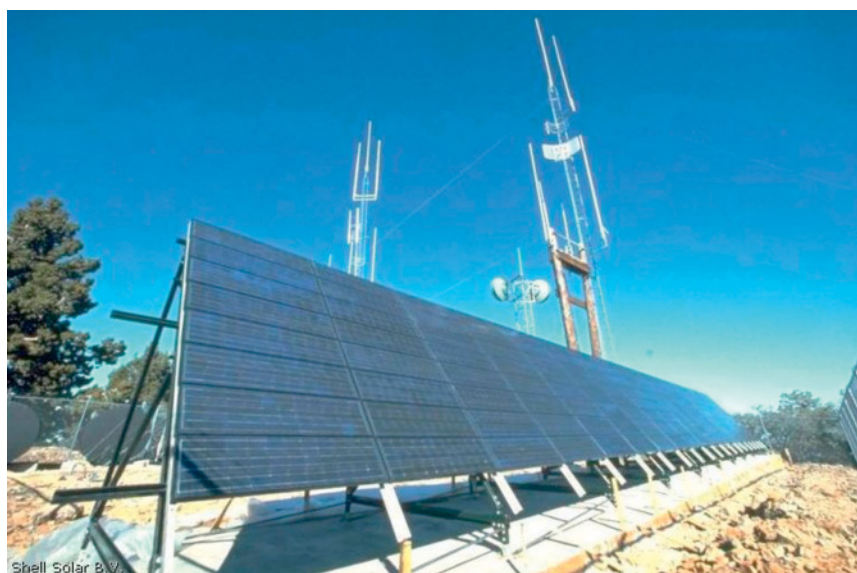
Figure 5.37 Another example of a large PV array in a remote location: this one helps to transmit information by telecommunications link (EPIA/Shell Solar).
