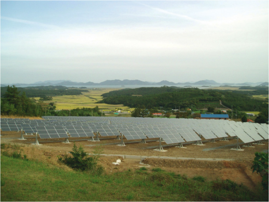
Figure 4.3 This Korean power plant uses four 250kW p inverters to connect 1MW p of PV arrays to the grid. The nonconcentrating modules are mounted on horizontal single-axis trackers (IEA-PVPS).
