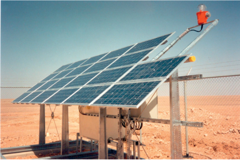
Figure 5.34 This installation in the Libyan desert provides cathodic protection , an important application of PV that helps minimise corrosion of metal structures including pipelines (EPIA/Shell Solar).
