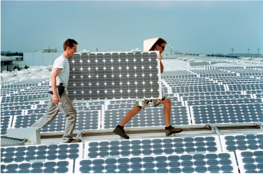
Figure 2.1 Each of these PV modules contains 72 monocrystalline silicon solar cells (EPIA/Phoenix Sonnenstrom).
