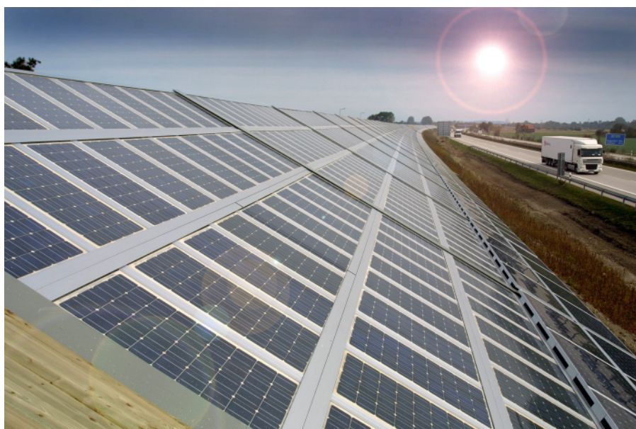
Figure 4.20 A 1.6km PV array gives added purpose to a highway sound barrier in Germany (EPIA/Isofoton).
