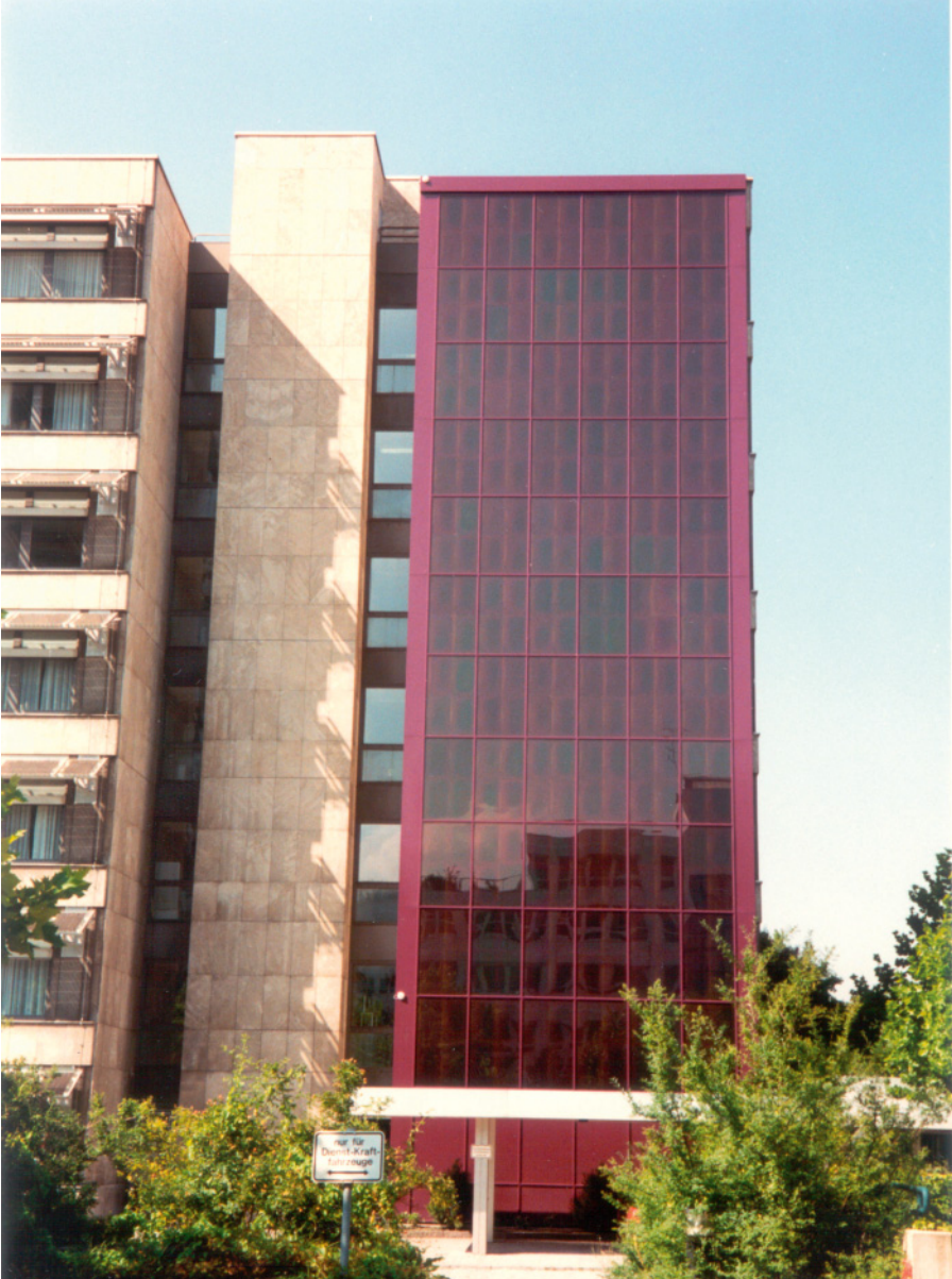
Figure 2.23 Amorphous silicon PV modules on a building façade (EPIA/Schott Solar).
