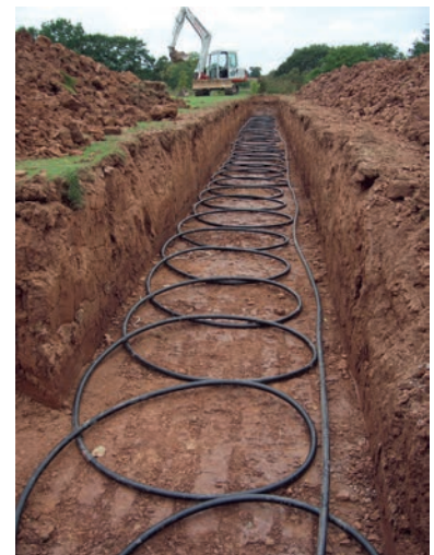
▲ Figure 1.15 Slinkies being installed in the ground
