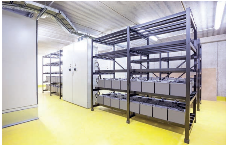
▲ Figure 7.12 Many single computers and installations have uninterruptable power supplies, so that they may be live even if the mains power is off
