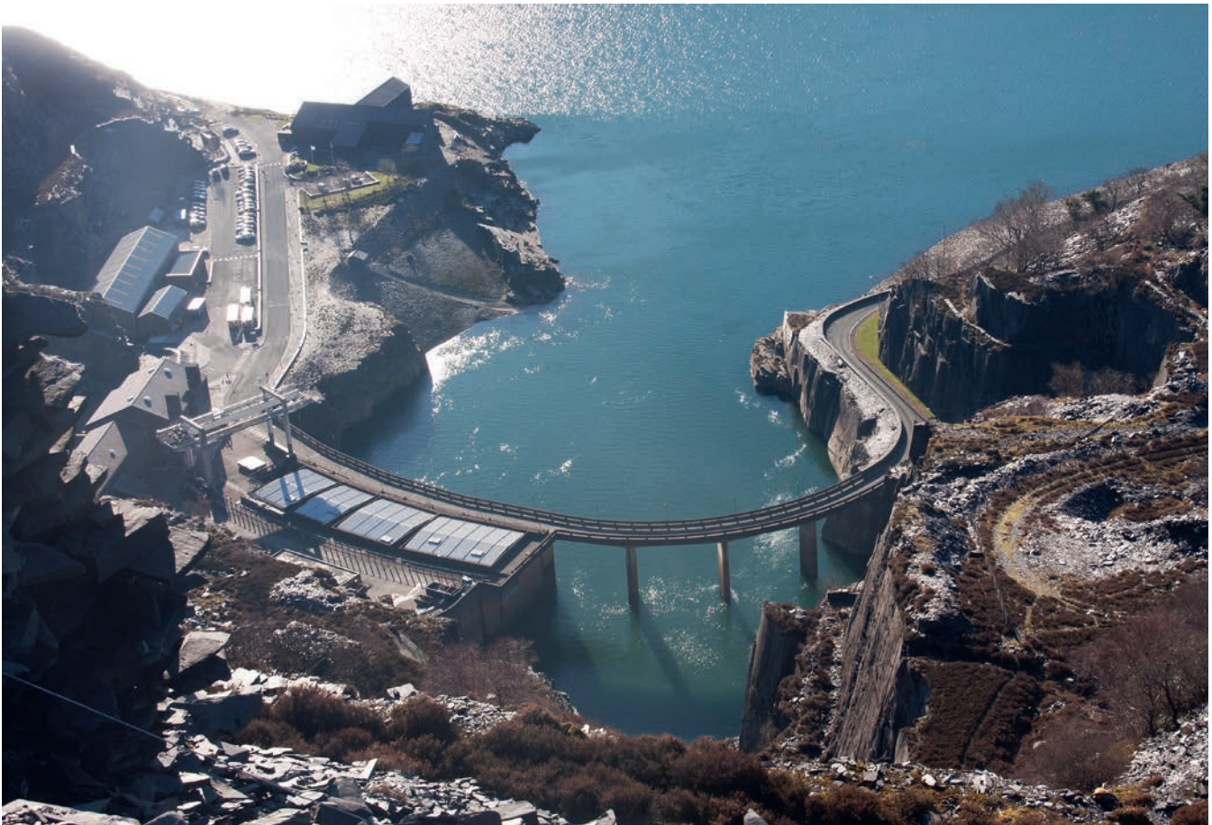
▲ Figure 2.5 Dinorwig (North Wales) pumped storage electricity generation scheme
