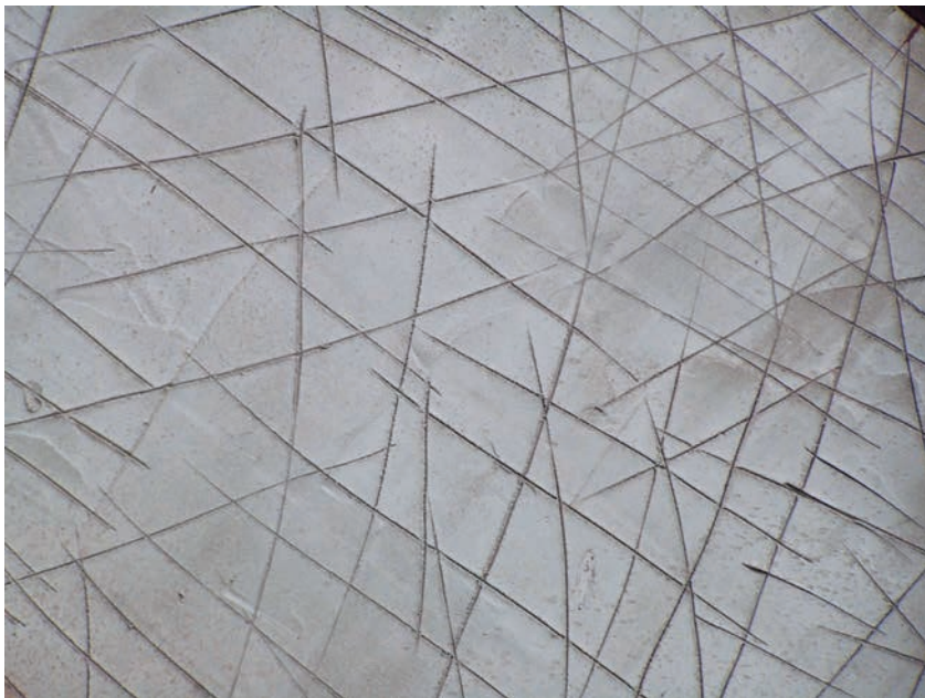
▲ Figure 4.13 Criss-crossed plaster
