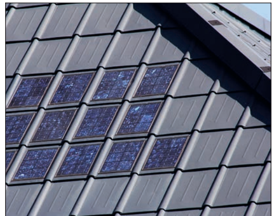
▲ Figure 1.24 In-roof mounted system
