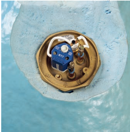
▲ Figure 2.126 Thermostat inside pocket in heater element
