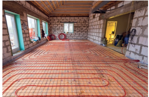
▲ Figure 2.120 Electric underfloor heating before the final screed is laid
