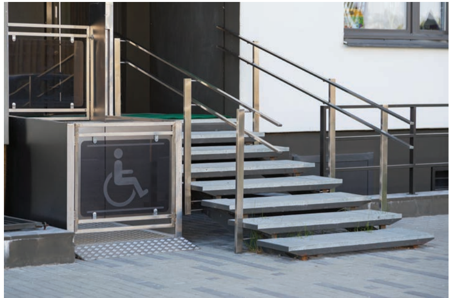
▲ Figure 5.16 Building entrance equipped with special lifting platform for wheelchair users
