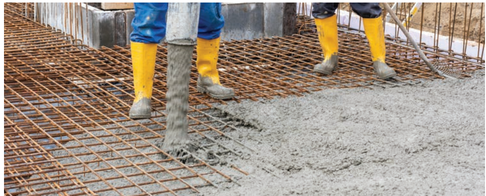
▲ Figure 3.22 Concrete being poured onto rebars to form a building foundation
