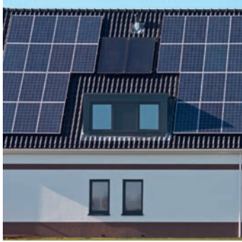
▲ Figure 1.29 Building features shading a photovoltaic system
