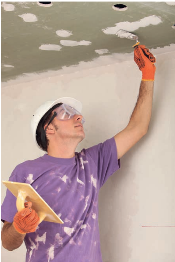
▲ Figure 4.14 Repairing a hole in plasterboard
