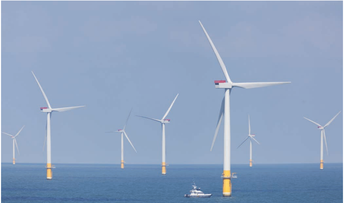
▲ Figure 2.6 A typical offshore wind farm installation
