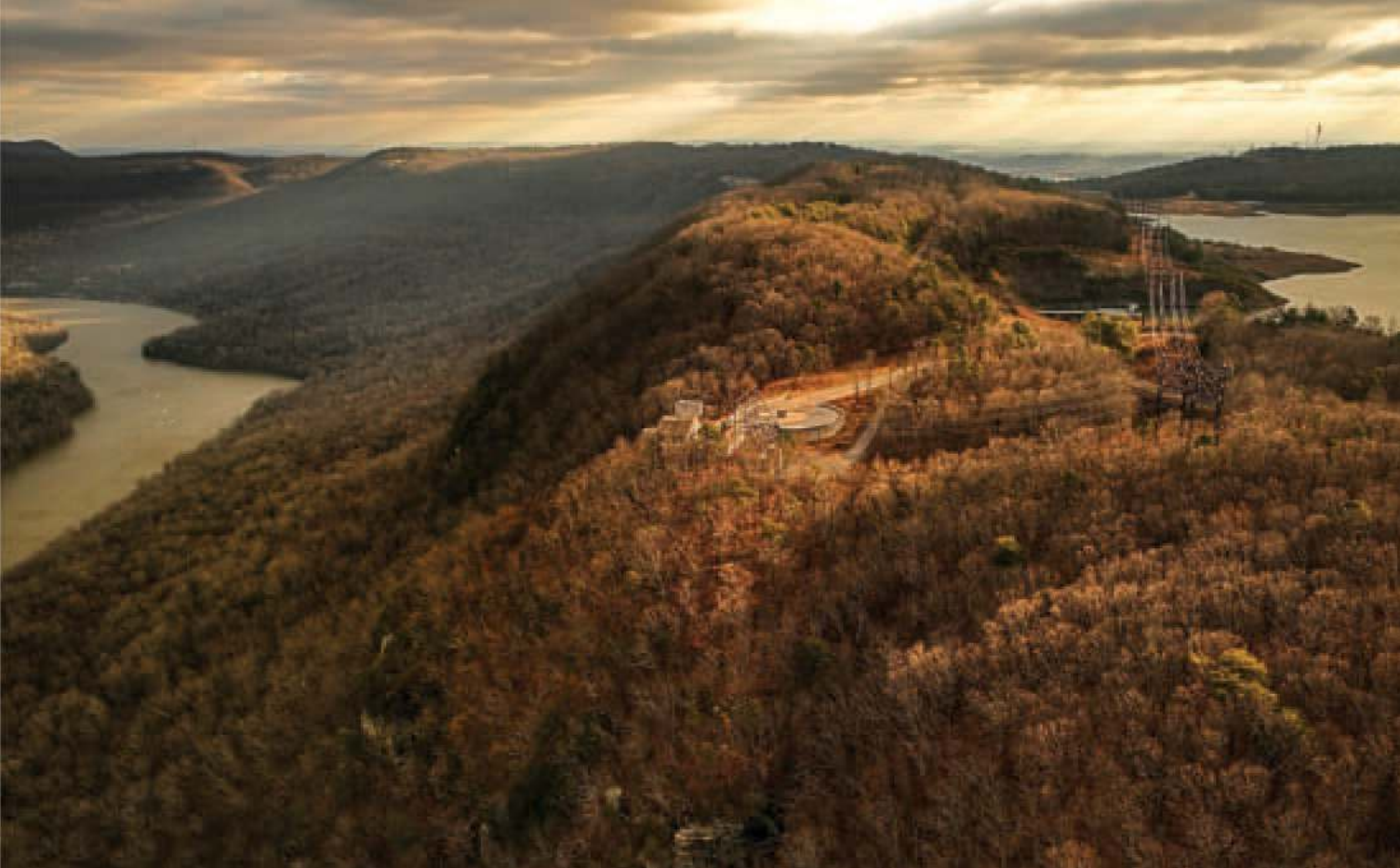
At Raccoon Mountain, west of Chattanooga, Tennessee, the upper reservoir is some 300 meters above the Tennessee River (left). The powerhouse is under the mountain.
