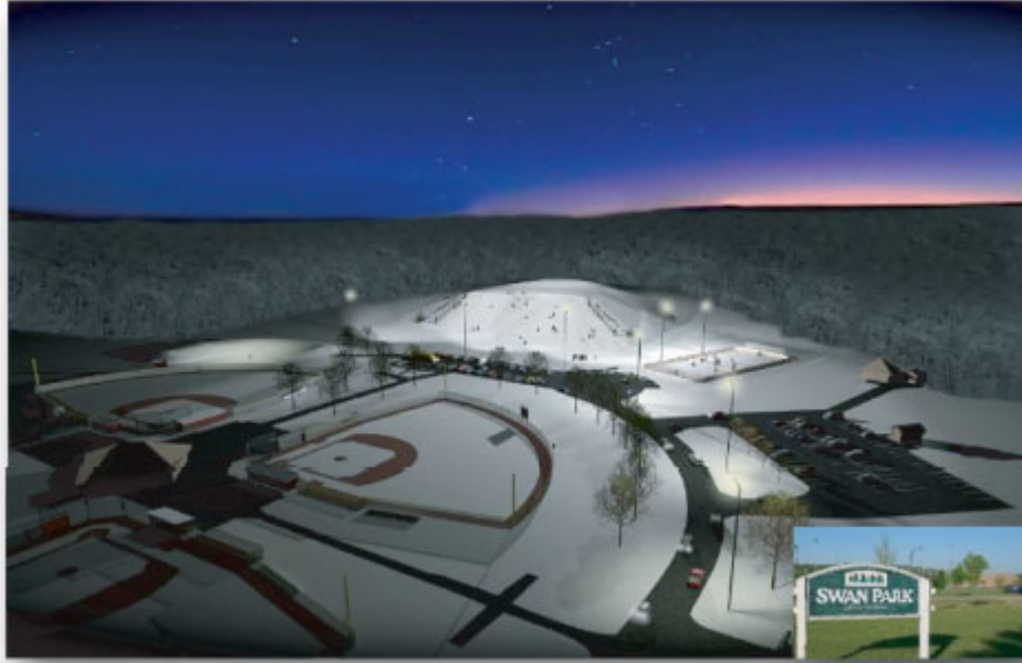
Figure 22.7 Foundry sand reuse for 42' sledding hill in Swan Park, Waupaca, WI.
