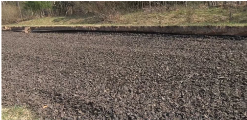
Figure 46.8 6 inches of tire-derived aggregate in Clare County construction.
