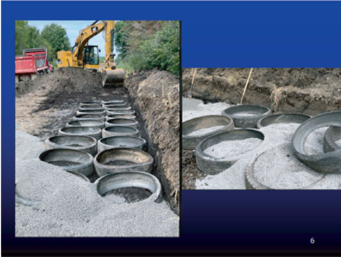
Figure 46.10 Tire-derived aggregate in Ingham County construction.
