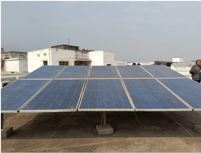
Figure 9.1 5-kW roof top solar plants.
