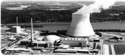
Attacks on Siemens PLCs paralyzed a nuclear plant.
