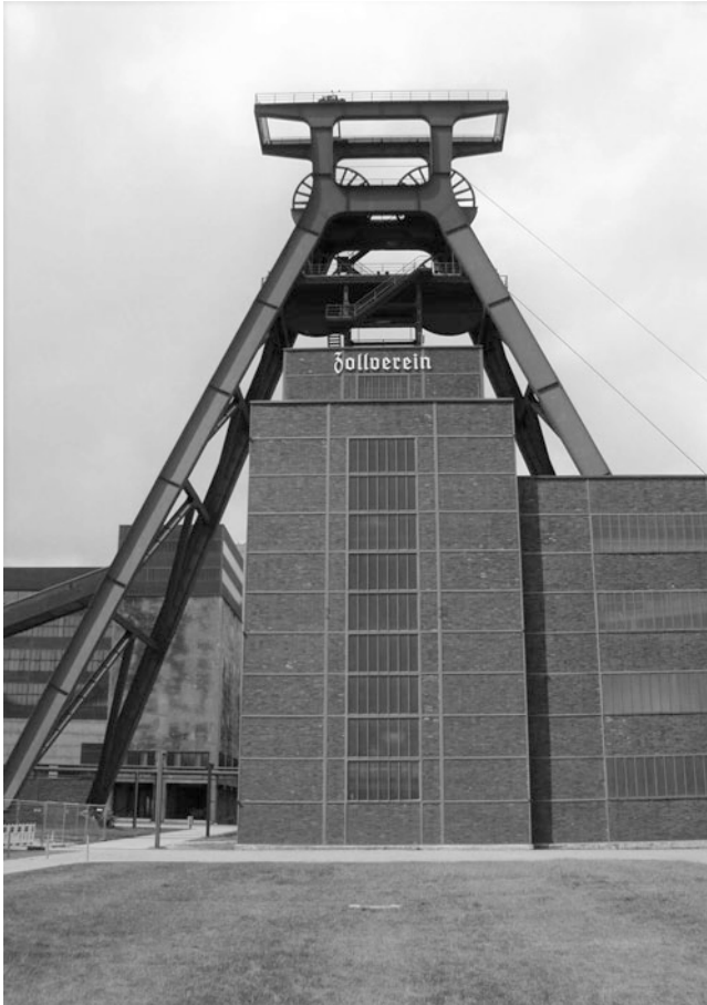
Fig. 8.1 The iconic steel hoisting frame over Zollverein's central Shaft XII. This hoisting frame was used to raise and lower conveyances within the mine shaft to transport coal, which was later sent to the coal washing plant where it was separated from rocks and other unwanted material. Although the mine ceased production in the 1986, the hoist is still used to pump water out of the empty mine shafts. Picture by the author (2014)
