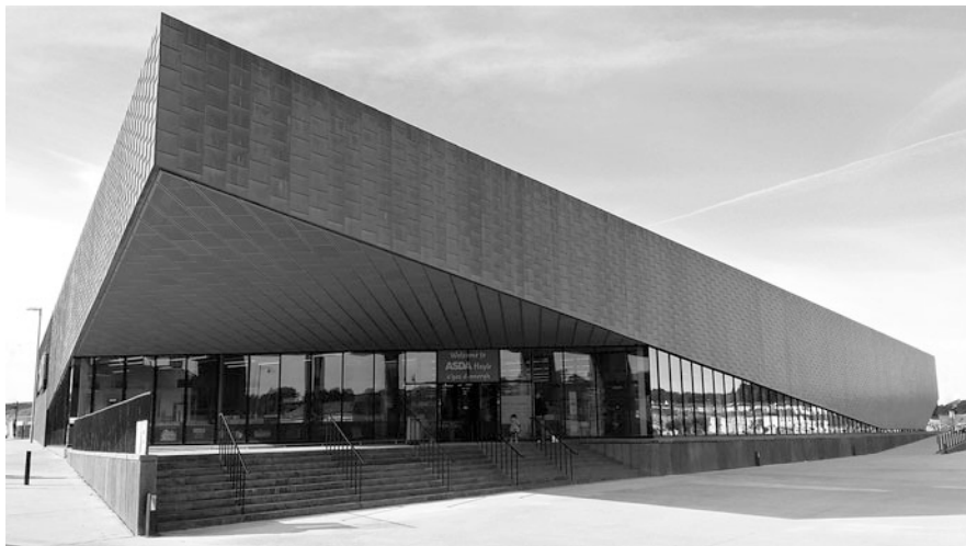
Fig. 9.4 The ASDA store in Hayle. According to the architects, this building was inspired by the mining history of Hayle. Copper cladding was used to cover the facades as a reference to the region's copper producing and manufacturing history. Picture by the author (2015)
