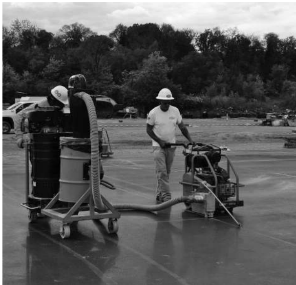
FIGURE 15.8 Cutting joints with an early-entry saw. The saw cuts dry, so a vacuum tags along to collect dust.
