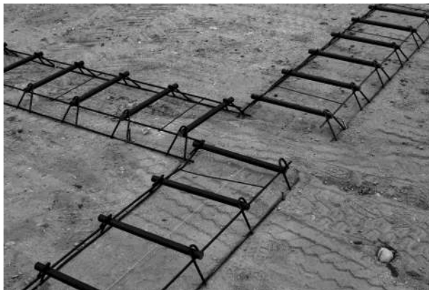
FIGURE 15.4 Round dowels at sawn joints. The wire frames holding the dowels are called baskets or cradles. On this job, the contractor marked the joint lines with taut string and nailed down the baskets. Most contractors aren't that careful.
