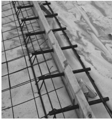
FIGURE 15.3 Round dowels at a construction joint.
