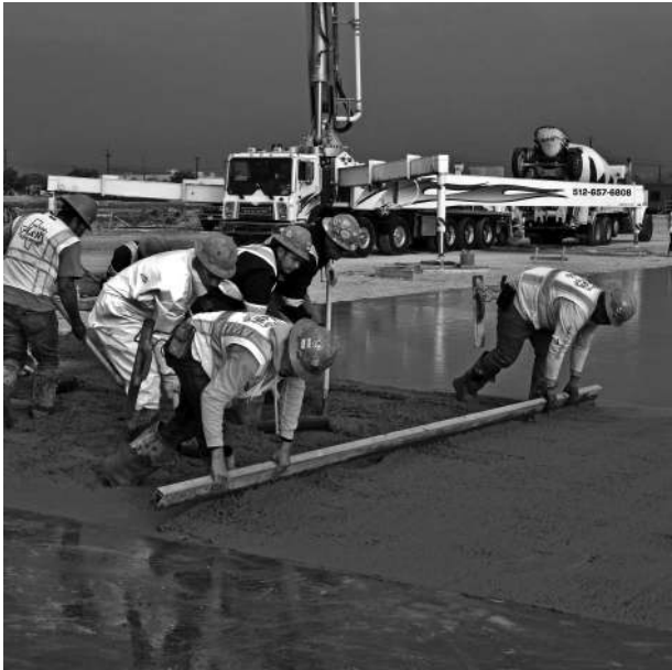
FIGURE 18.1 Striking off with a hand straightedge.
