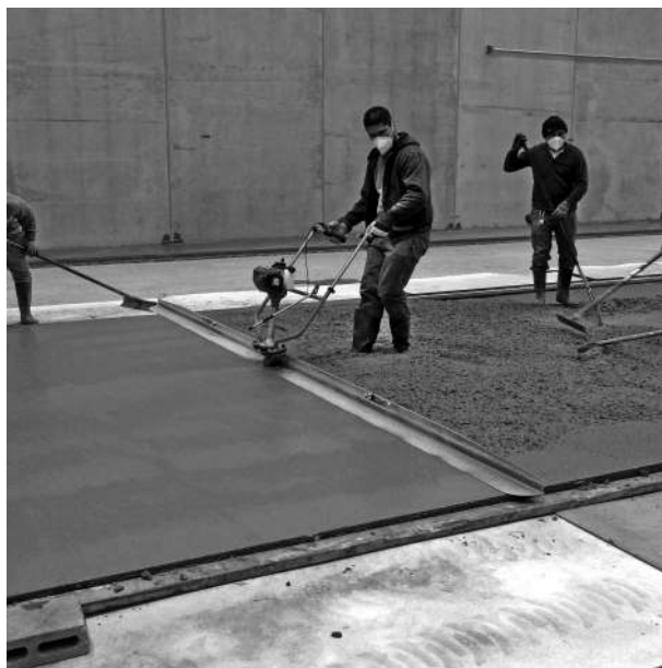
FIGURE 18.3 A wet-screed vibrator, used here on a narrow-strip pour.
