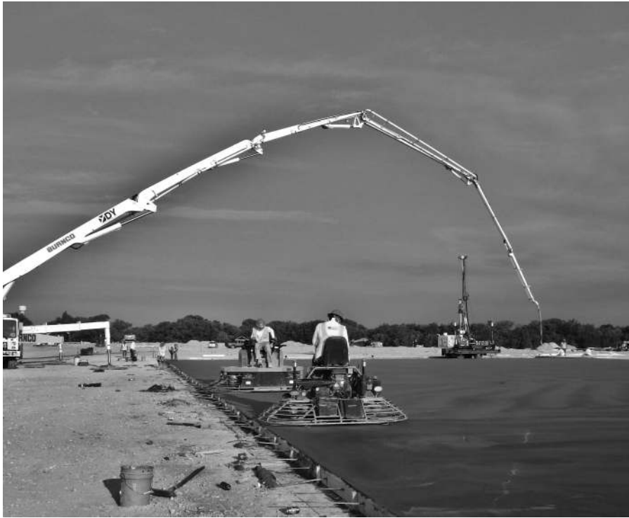
FIGURE 10.2 Boom pumps work well outdoors and can be used indoors too on some warehouse jobs.
