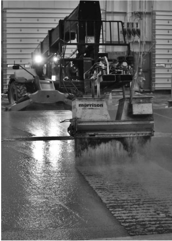
FIGURE 18.13 A metallic shake being dropped from a power spreader.
