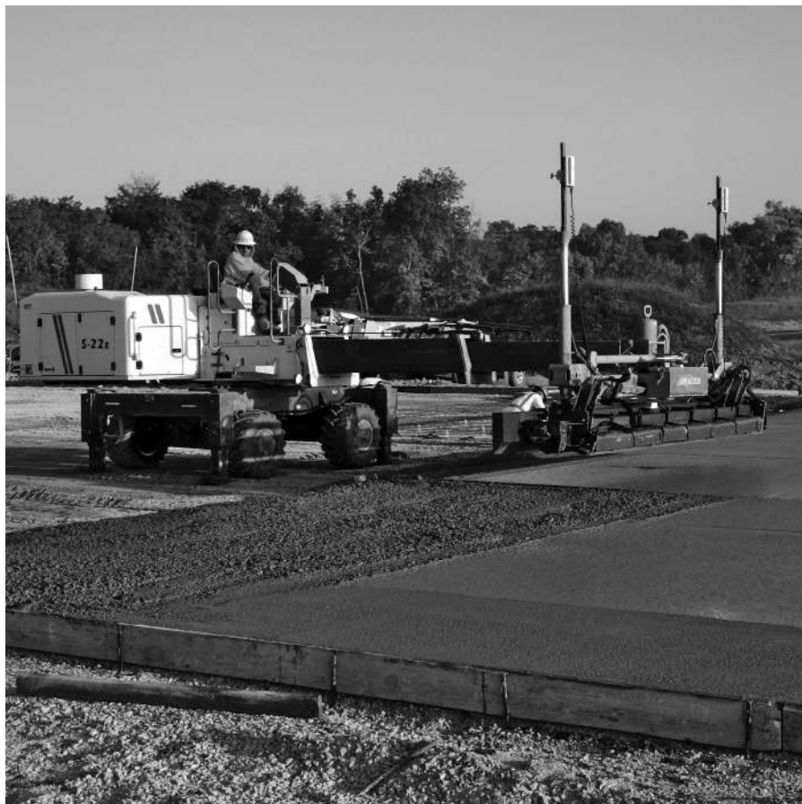
FIGURE 18.5 A laser screed on a large-bay pour.
