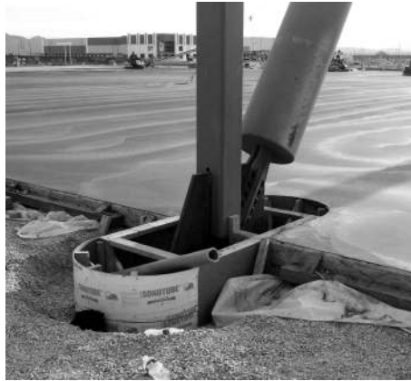
FIGURE 15.2 Columns of unusual shape call for special blockouts, with forms constructed on site. This type is called a hockey-rink blockout because of its shape.
