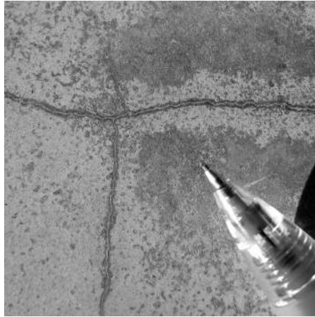
FIGURE 13.2 Crazing as mild as this is harmless and should be ignored. But see Figure 13.3.
