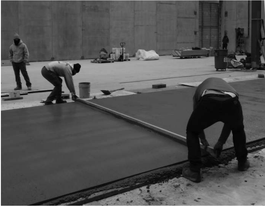
FIGURE 20.7 Reworking a superflat pour with a hand straightedge.
