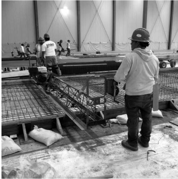
FIGURE 18.4 A truss screed.
