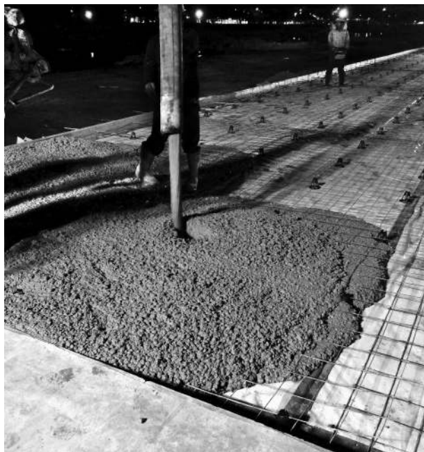
FIGURE 6.4 A highly finishable concrete mix.
