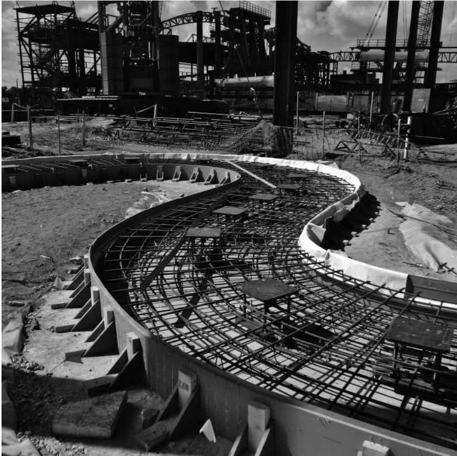
FIGURE 20.6 An unusual superflat floor, laid for an amusement park ride.
