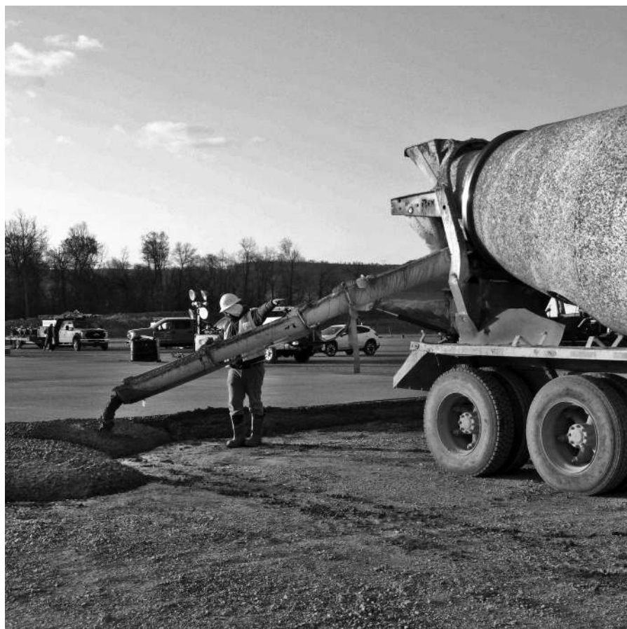
FIGURE 10.1 Tailgating, or pouring directly from the concrete truck into the forms, is the simplest way to place concrete.
