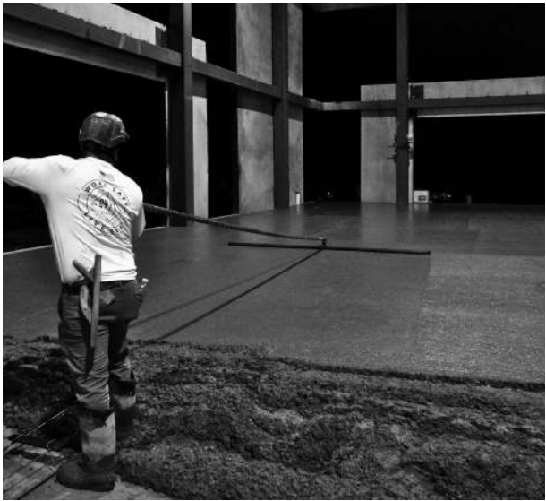
FIGURE 18.2 A lightweight highway straightedge, also called a check rod, on a large-bay pour.
