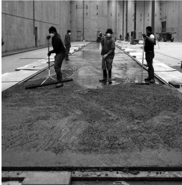
FIGURE 19.2 A bonded topping under construction.
