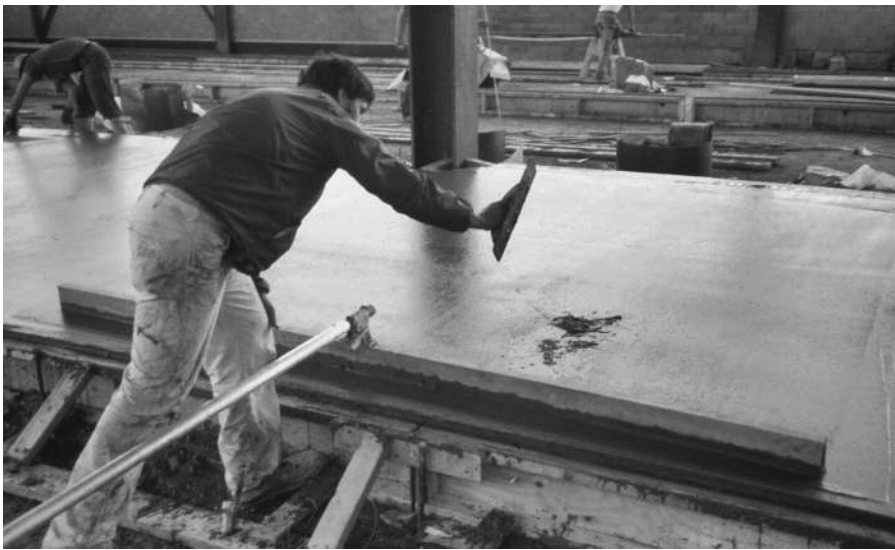
FIGURE 20.8 This worker has just scraped the floor with a highway straightedge and is about to add mortar to a low spot.
