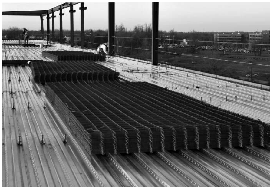
FIGURE 5.7 Composite slab under construction in an office building. The corrugated steel deck is both soffit form and bottom reinforcement. The wire mesh will be laid in a single layer to control shrinkage cracks. Note the shear studs, like big nails, sticking up in rows. They provide composite action between the slab and the structural steel frame.
