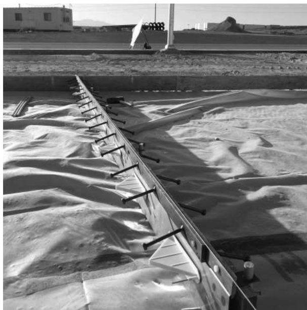
FIGURE 15.10 An armoured joint, ready for concrete to be poured.
