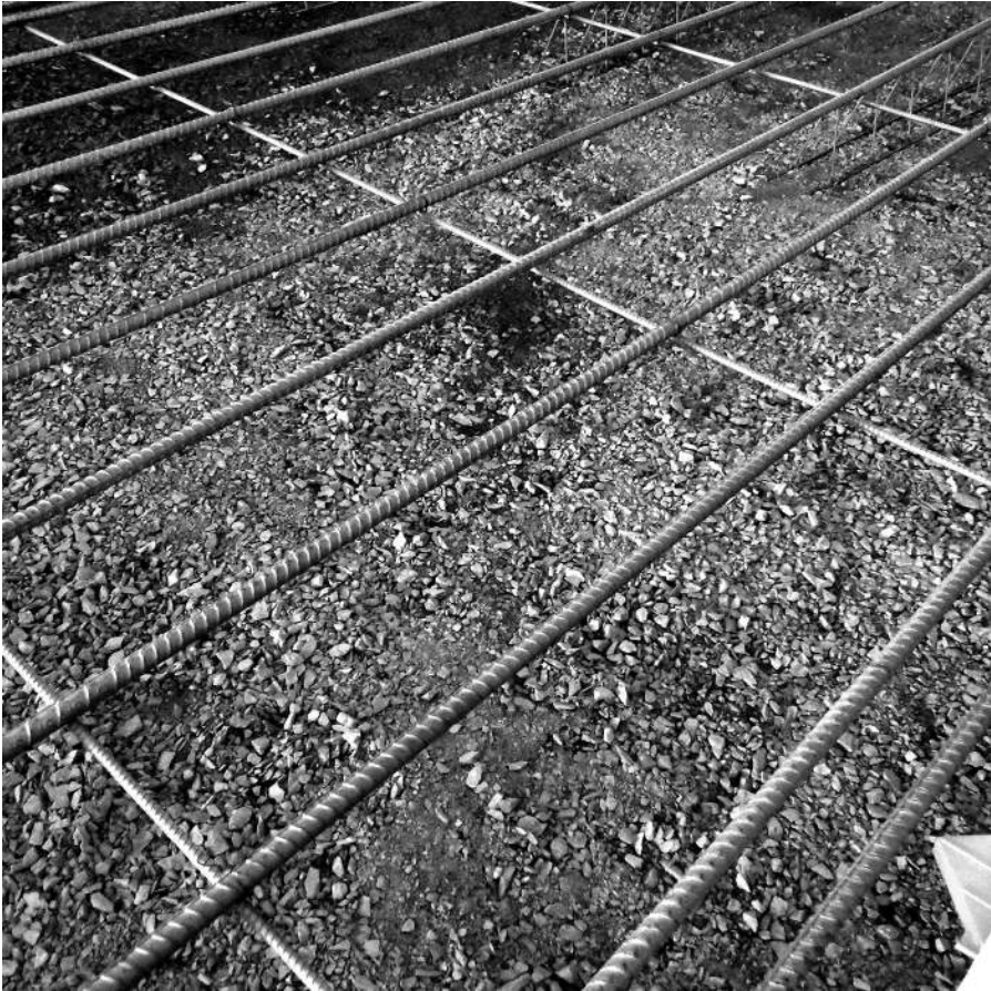
FIGURE 16.2 One-way reinforcement in a narrow-strip superflat slab.
