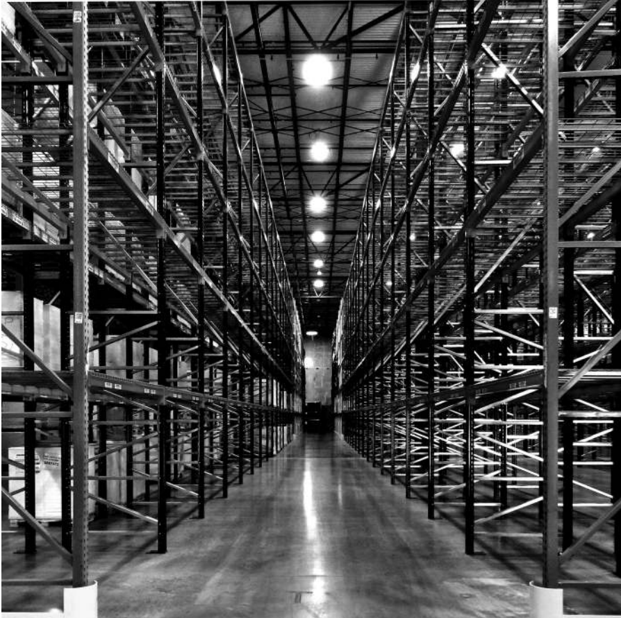
FIGURE 2.2 Pallet racks. This is a very common configuration, with beams that hold two pallets side by side, and with the bottom pallets resting on the floor.
