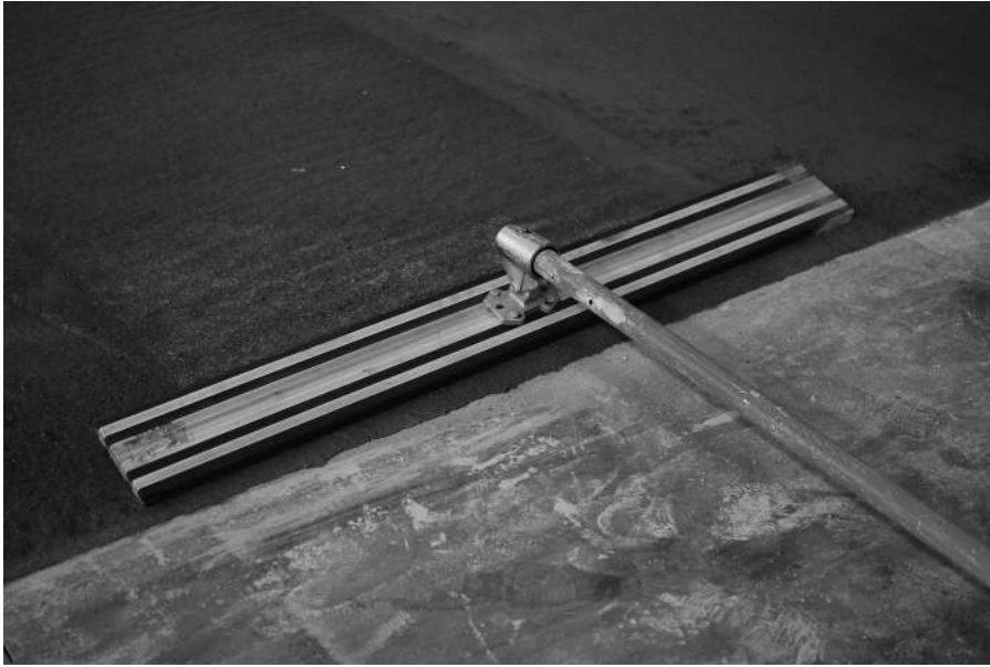
FIGURE 18.6 A bull float with a blade of laminated wood being used on a dry shake.
