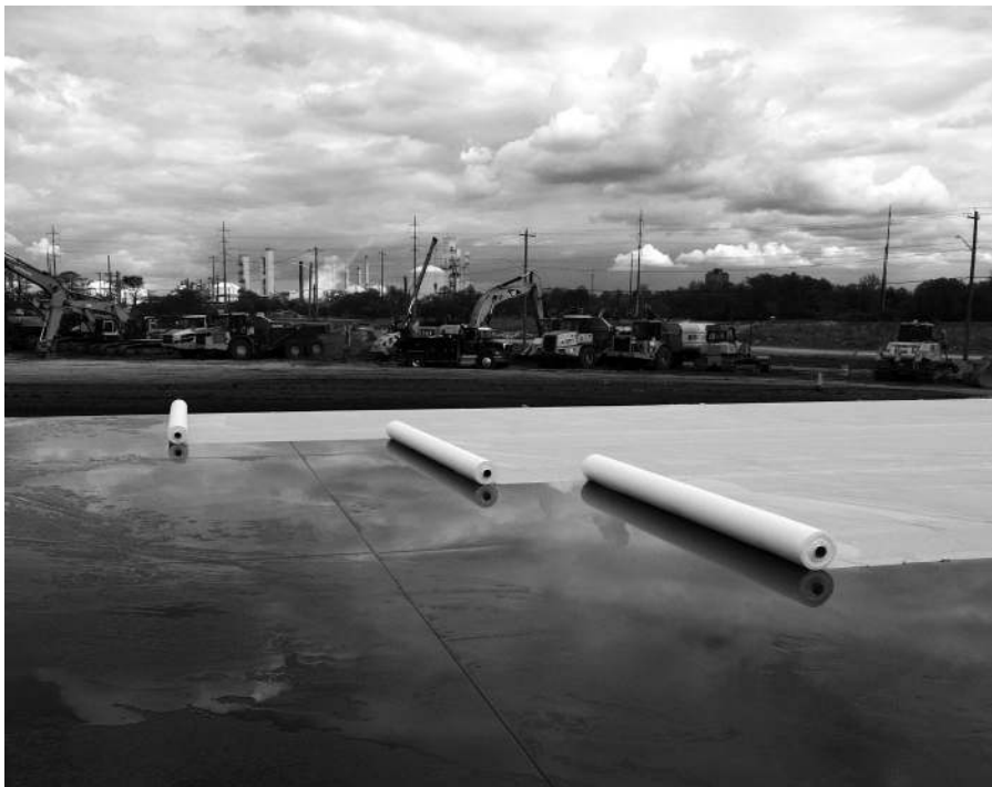
FIGURE 11.1 Curing with impervious sheet material.
