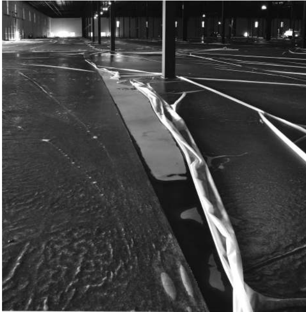
FIGURE 11.2 Dry spots like this should be soaked and recovered right away.
