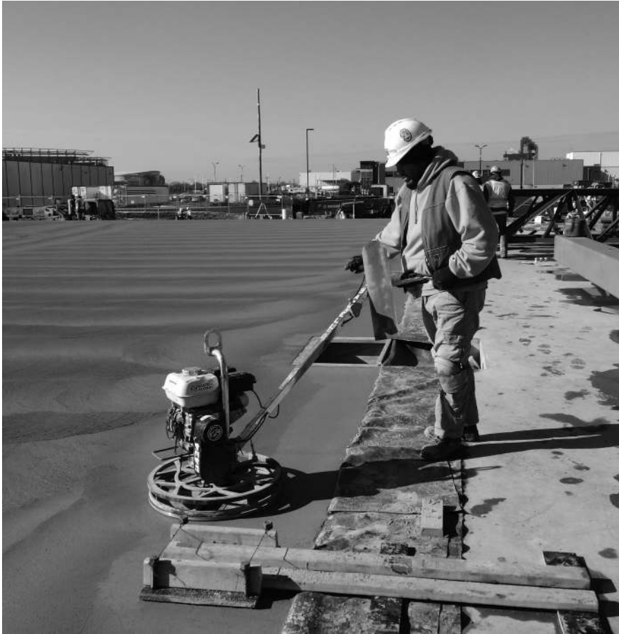
FIGURE 18.9 A small walk-behind trowel machine used at an edge. Most walk-behinds are bigger.
