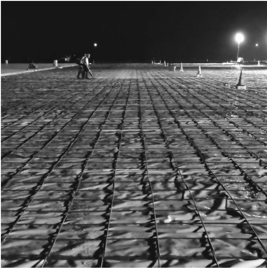
FIGURE 16.3 Reinforcement for enhanced aggregate interlock, with 0.1% steel in two directions. The mat will be raised during the pour and supported on plastic chairs.
