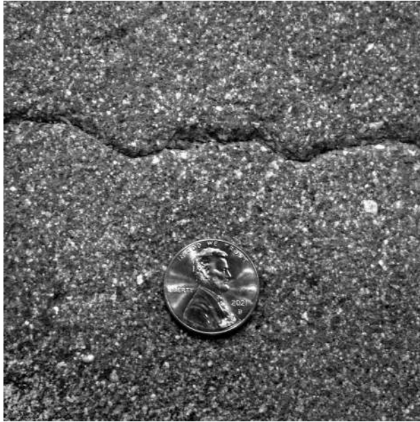
FIGURE 22.2 A surface prepared by shot-blasting.
