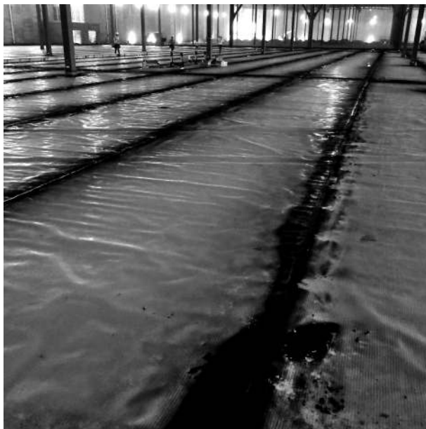
FIGURE 22.1 Heavy-duty vapour barrier with sealed seams, on a brownfield site.
