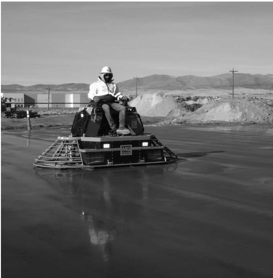
FIGURE 18.8 A ride-on trowel machine with finish blades.
