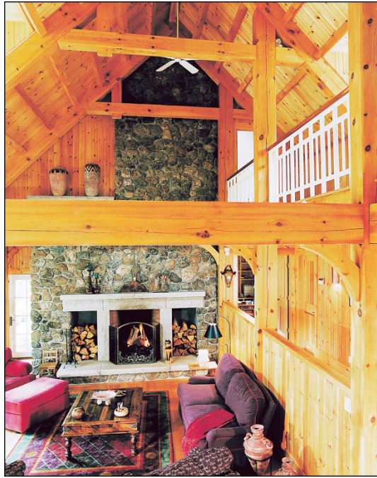
FIGURE 4-2: The beauty of wood timbers is revealed in the home's interior, where posts and beams allow for open, vaulted spaces.
