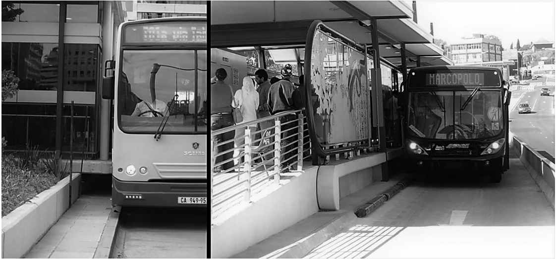
FIGURE 10.19 Kassel kerbs in Cape Town (left) and alignment markings in Johannesburg (right)
