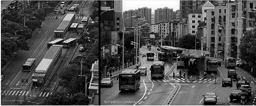
FIGURE 10.17 Bus rapid transit stations with dual-side docking for buses in a single direction
