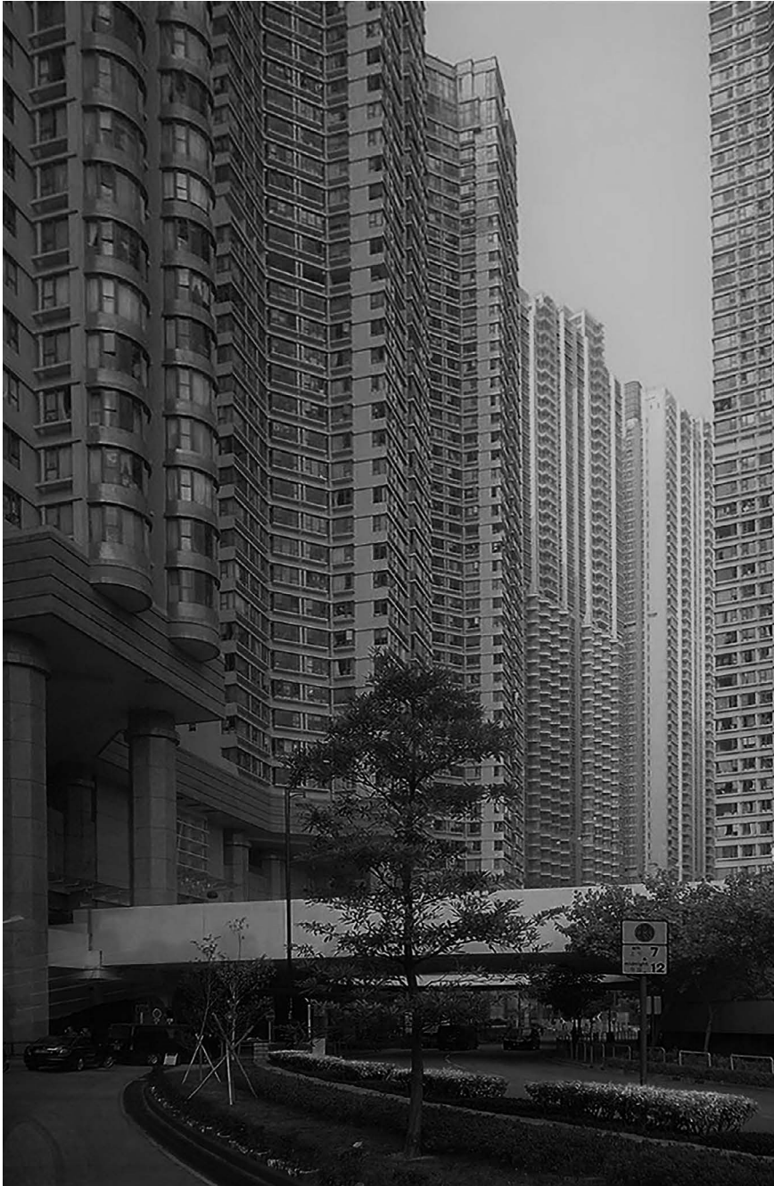
FIGURE 8.5 High-rise wall in Hong Kong
