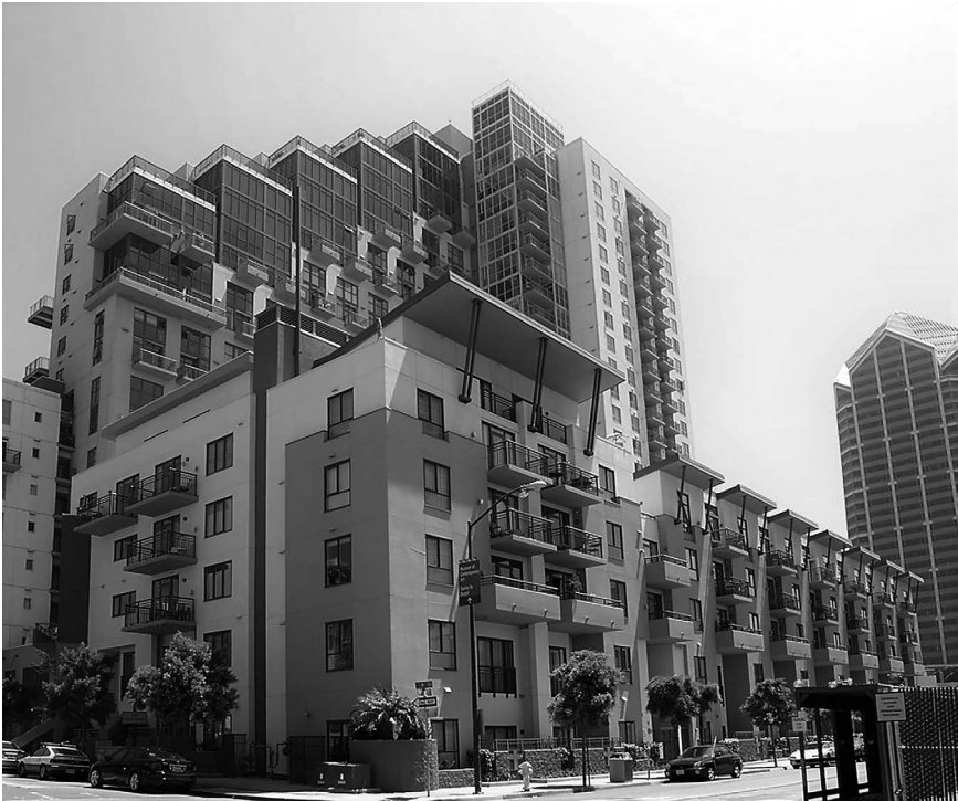
FIGURE 8.13 Downtown San Diego: the high-rise slab is arranged back to back with mid-rise stacked flats within the same block. This block type is particularly suited along corridors to transition high densities into adjacent lower density fabrics
