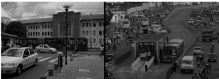
FIGURE 10.15 Median busways alignment avoids conflicts Ecovia, Quito, Ecuador (left) and Rainbow, Pune (right)
