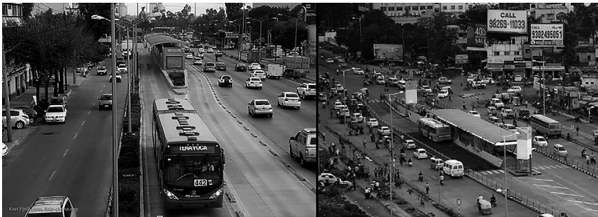
FIGURE 10.13 A single-lane bus rapid transit system in Mexico City (left)
