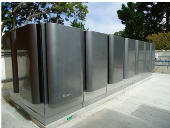
Fig. 9.29 Installation of “Bloom Box” solid oxide high temperature natural gas fuel cells produced by Bloom Energy (USA) circa 2015. Photo from Wikipedia Commons. 9 March 2020 https://commons.wikimedia.org/wiki/Category:Bloom_Energy_Server . Attribution CC BY 2.0
