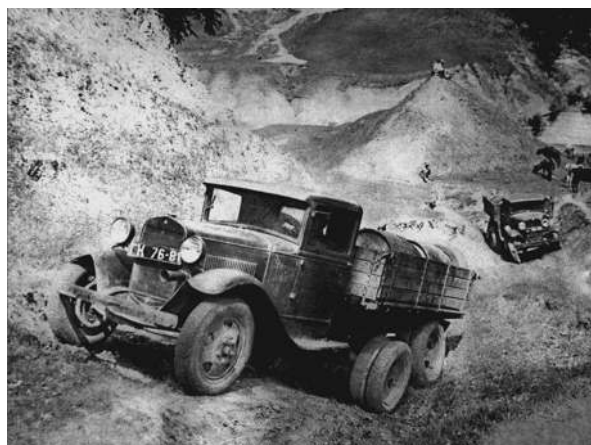
Fig. 9.6 Russian hydrogen powered GAZ-AAA truck, 1941. From Hydrogen Cars Now, “Tense Times in Hydrogen and Fuel Cell History” 28 June 2017 https://www.hydrogencarsnow.com/index.php/history/tense-times-in-hydrogen-and-fuel-cell-history/ Article copyright George Wand. Historical image public domain
