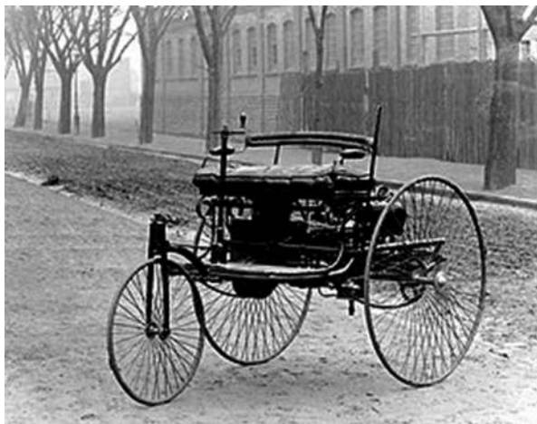
Fig. 3.1 Benz Motorwagen, 1886, Germany, which is considered the first successful automobile, constructed by Rheinische Gasmotorenfabrik Benz & Cie. (Mercedes-Benz) Image from Deutsches Automotiv Museum, Munich DE. Public domain
