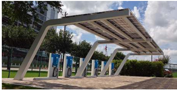
Fig. 14.83 Lumos Solar Canopy EV Charger installed at workplace. Image from https://lumossolar.com/2015714nrg-evgo-features-lsx-modules-at-nrg-stadium/img-jpg-41/ . With permission
