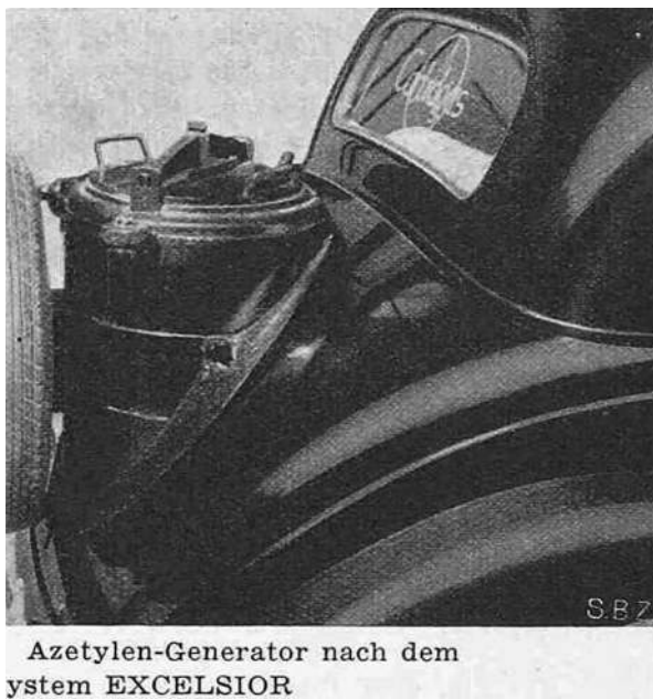
Fig. 16.11 Calcium carbide acetylene gas generator built into trunk (boot) of a passenger sedan, circa 1930, Germany. Image public domain, from museum archive. http://www.douglas-self.com/MUSEUM/POWER/acetylene-eng/excelsior2.jpg
