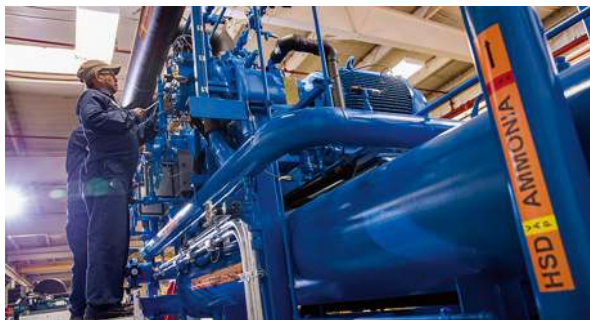
Fig. 10.5 Industrial food storage refrigeration apparatus. From 2023 Berg Chilling Systems Inc., https://berg-group.com/blog/food-and-beverage/refrigeration-equipment-food-beverage/ . With permission
