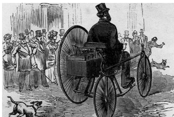
Fig. 14.2 Electric-assisted pedal trike built by inventor Gustave Pierre Trouvé, demonstrated at the Paris Electric Exhibition April 1881. Novel but dangerous power control involved raising and lowering lead plates in the sulfuric acid battery electrolyte (seen behind the driver). Image from Scientific American , pre-1800, public domain, as included in History of the Electric Automobile , Ernest Wakefield, SAE Publication, 1994
