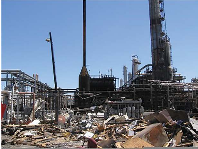
Figure 24.8 Photo of the blowdown unit of BP Texas City Refinery (Source: US Chemical Safety board, www.csb.gov ).
