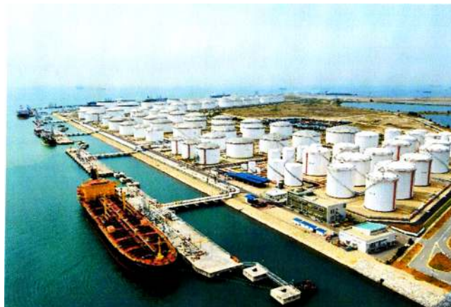
Figure 25.1a Refinery tank farm blending and shipping facilities.
