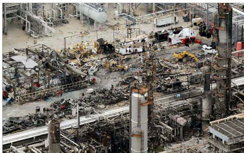
Figure 24.2 Photo of BP Texas City, TX Refinery after the explosion (Source: www.csb.gov).
