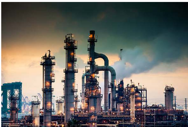
Figure 26 A photo of petroleum crude oil refinery.
