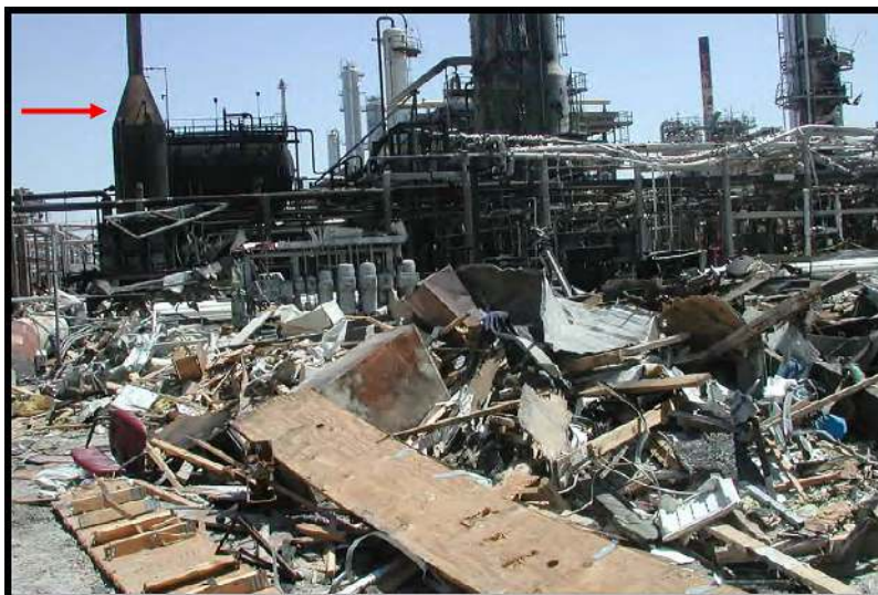
Figure 24.3 Photo of destroyed trailers west of the blowdown drum (red arrow in upper left of the figure, www.csb.gov ).
