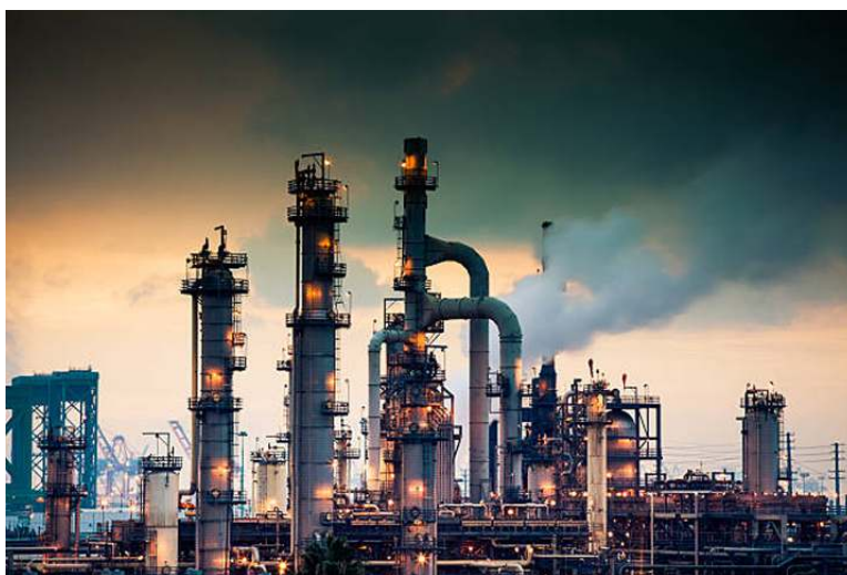
Figure 26 A photo of petroleum crude oil refinery.
