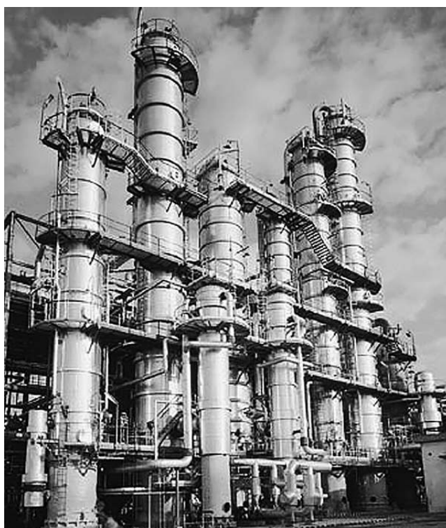
Figure 19.2a A photograph of fractionating columns showing De-methanizer, De-ethanizer, De-propanizer, and De-butanizer units (courtesy of Sulzer Chemtech Ltd.).
