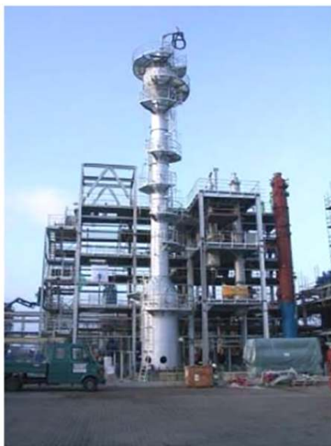
Figure 20.98A A photo of liquid–liquid extraction column for aromatic purification (source: Koch Modular Process System (KMPS) LLC).
