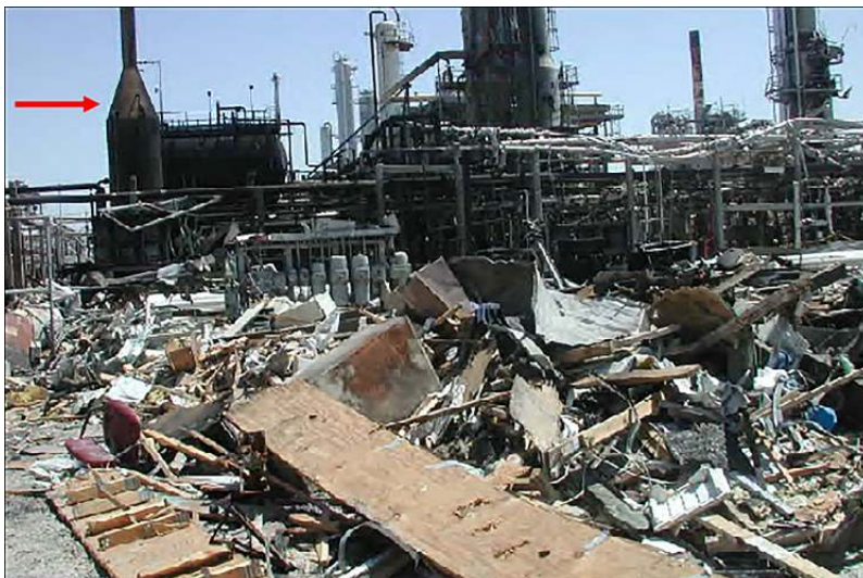
Figure 19.204 Portable buildings destroyed where contractors were located west of the blowdown drum (red arrow in upper left of the figure) (Source: www.csb.gov ).
