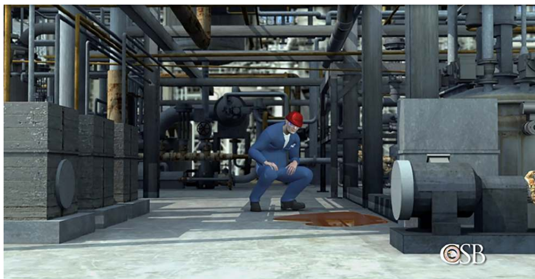
Figure 19.208 CSB animation depicting operator identifying the leaking 4-sidecut pipe (Source: www.csb.gov).
