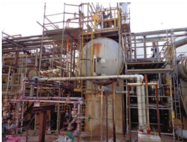
Figure 10.23 Photograph of DCRC Alkylation unit during maintenance (Source: csb.gov)
