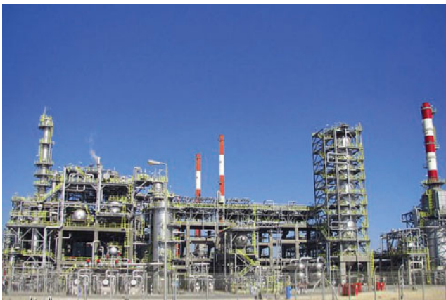
Figure 12.5 A typical Ultra-low-sulfur diesel unit (ULSD), with a fixed-bed reactor on the right.
