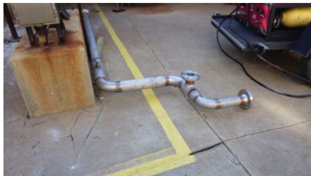
Figure 10.15 20-foot replacement piping (Source: csb.gov).
