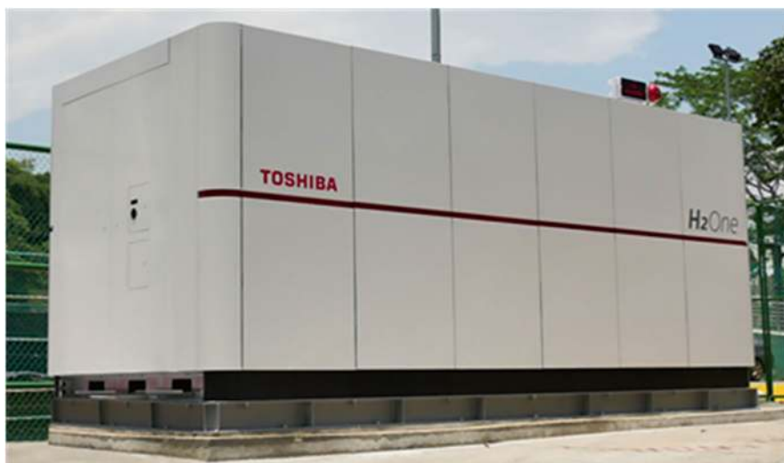
Fig. 5.23 The H 2 One “hydrogen production-hydrogen storage-power generation” integrated system
