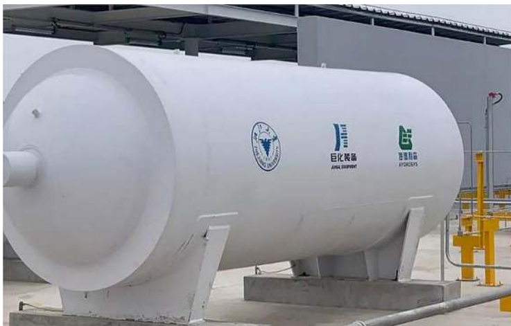
Fig 2.11 A steel strip mis-wound hydrogen storage container developed by Zhejiang University and Juhua Company
