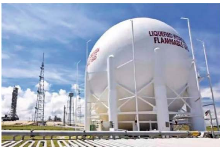
Fig. 3.7 A spherical liquid hydrogen storage tank insulated with vacuum glass microspheres by NASA, USA
